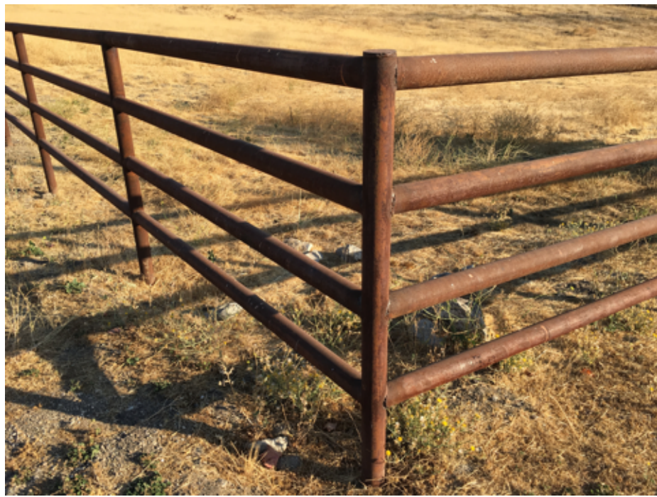
Existing 4'-6" Ht. Metal Pipe Fence
