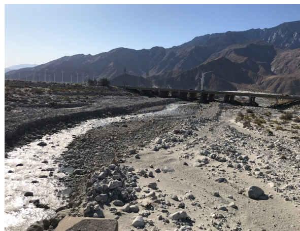
Colorado River water is conveyed along the 5-mile-long earthen channel, beneath I-10 to the Windy Point intake/sluicing structure.
