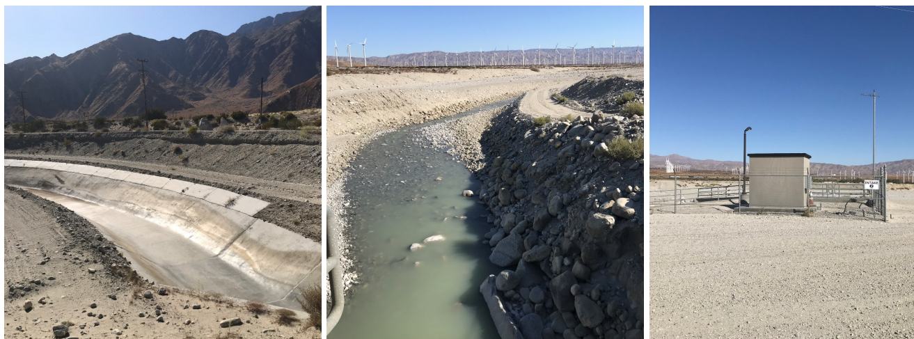
Depending on the flow and sediment load, water is delivered at the Windy Point intake/slucing structure to either be conveyed utilizing the cement-lined conveyance channel (left) and discharged directly into Ponds 1, 10, and 14 or diverted via an earthen channel (middle) to Intake Structures 1 and 2 (right), discharging to Ponds 1, 2, and 10.
