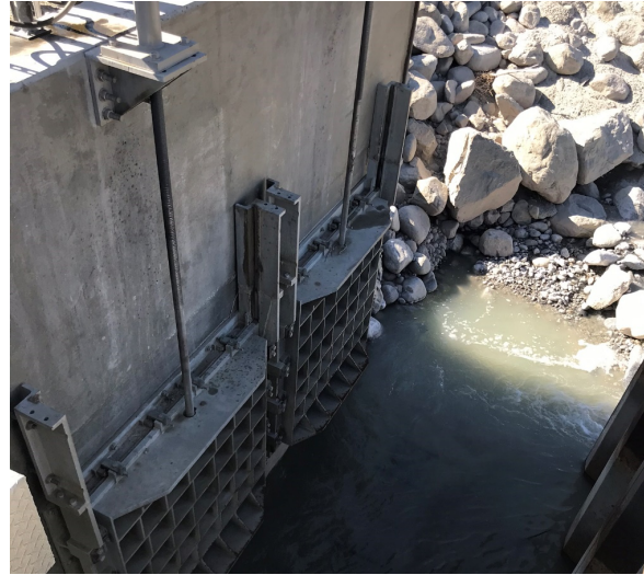
The Windy Point intake/sluicing structure is used to manage sediment loads in the water before it reaches the 19 replenishment ponds.
