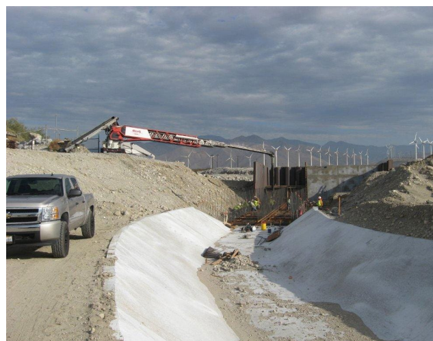
In 2013, CVWD completed construction of a new intake/sluicing structure and a 12,000-foot-long concrete-lined conveyance channel as well as groundwater replenishment pond improvements.
