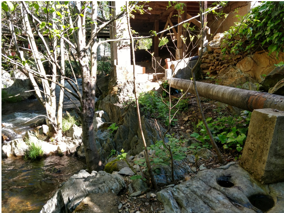
Photo 8. Photo taken of existing sewer line in Angels Creek near manhole #32A looking north. Existing sewer line is above ground in this segment.
