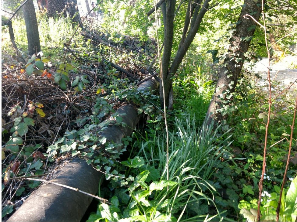
Photo 7. Photo taken of existing sewer line in Angels Creek near manhole #33 looking south. The existing sewer line is above ground in this segment.
