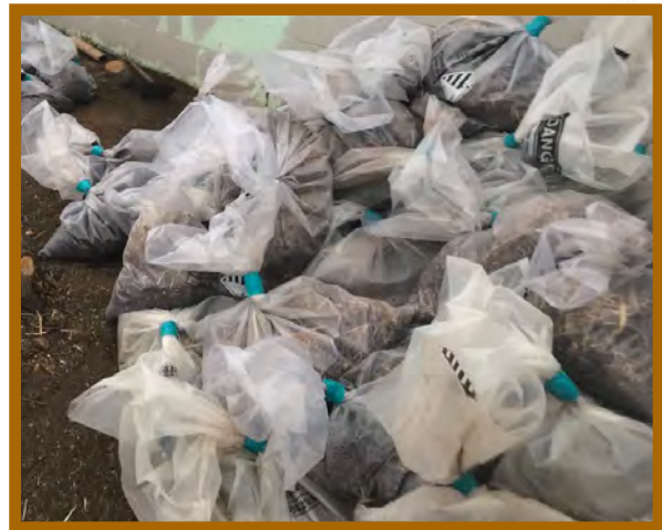
Contaminated Soil are bagged in Waste plastic asbestos bags
