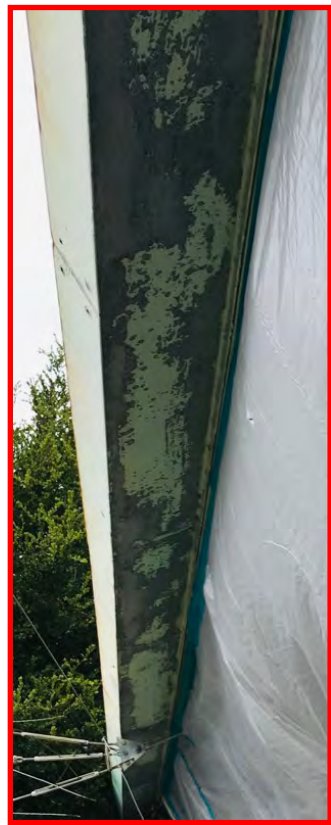
Exterior roof Eve Surface following Loose & Peeling Lead Based Paint removal & Stabilization in the Building C.
