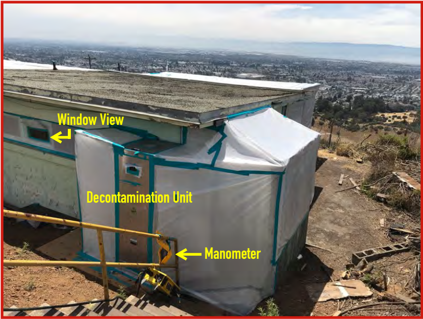
Building D, the decontamination unit & the negative air pressure
