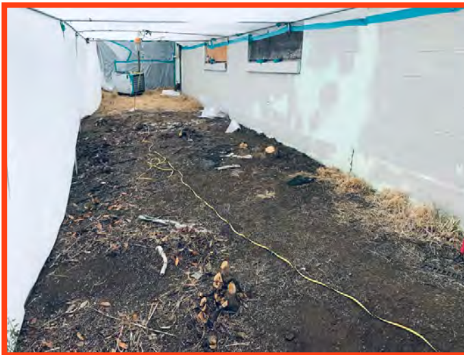
Before Contaminated Soil with ACM TSI Pipe Insulation debris clean up
