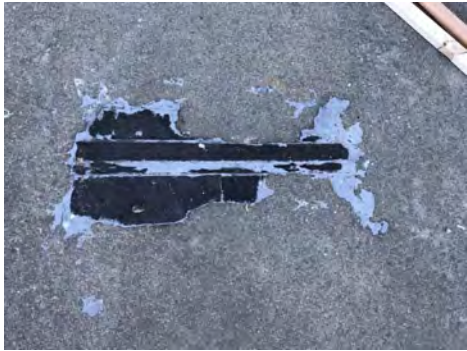
Remaining ACM Patching Compound on the Metal Duct & Concrete Flooring around the Bldg B Exterior.
