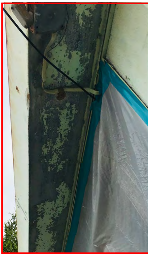
Exterior roof Eve Surface following Loose & Peeling Lead Based Paint removal & Stabilization in the Building C.
