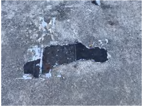
Remaining ACM Patching Compound on the Metal Duct & Concrete Flooring around the Bldg B Exterior.
