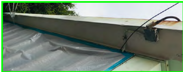
Exterior roof Eve Painting with primer following Loose & Peeling Lead Based Paint removal & Stabilization in the Building C.
