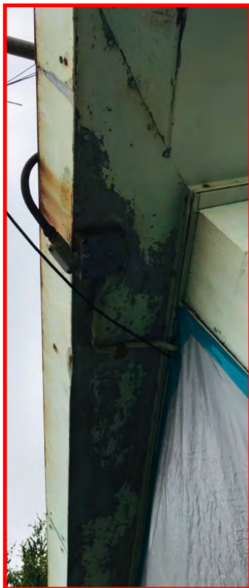
Exterior roof Eve Surface following Loose & Peeling Lead Based Paint removal & Stabilization in the Building C.
