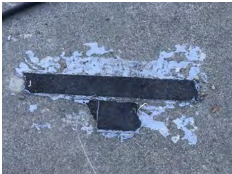
Remaining ACM Patching Compound on the Metal Duct & Concrete Flooring around the Bldg B Exterior.
