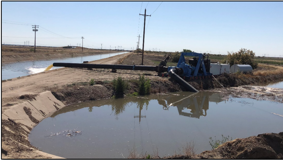
Figure 2-2: Existing Mobile Diesel-Powered Pumps at the Project Site
