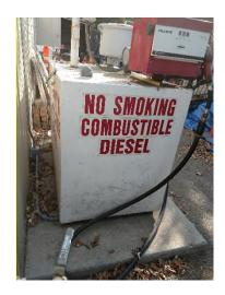
Figure 6 – View of 250-gallon diesel AST with alarm and double-wall containment.
