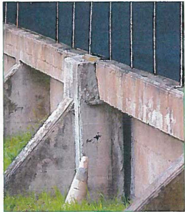
Figure 3 Damage to Reservoir Foundation in 2017 and 2019
