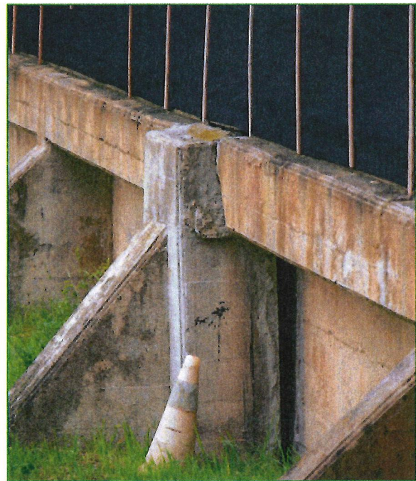
Figure 3 Damage to Reservoir Foundation in 2017 and 2019
