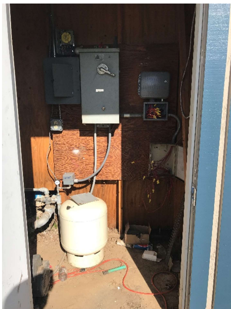
Photograph 23 – Photograph showing the pressure tank and control box for field irrigation. Equipment is housed in the storage shed on the northern border of the subject property
