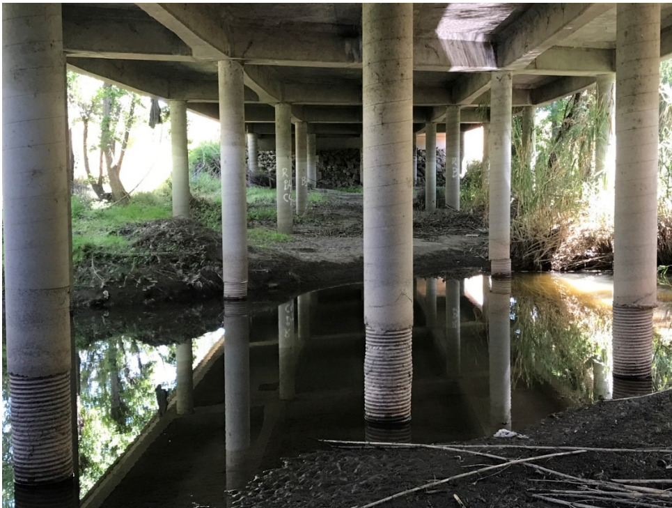
Figure 1-3 Mainline Exposed Bridge Piles
