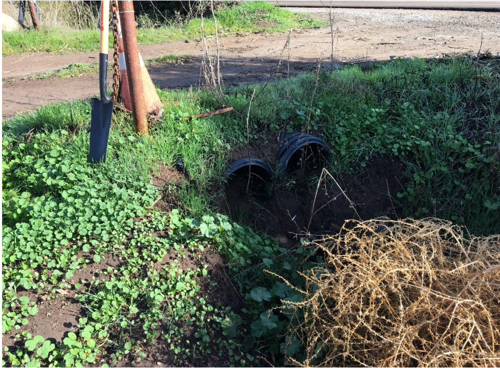
Ditch 1 – Close-up of culvert under the unpaved access road to the site.
