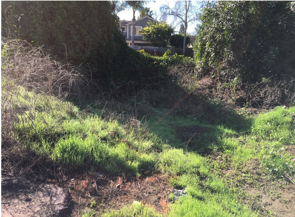
Ditch 1 – Downstream terminus of drainage. Note: lack of connectivity to Drain 1
