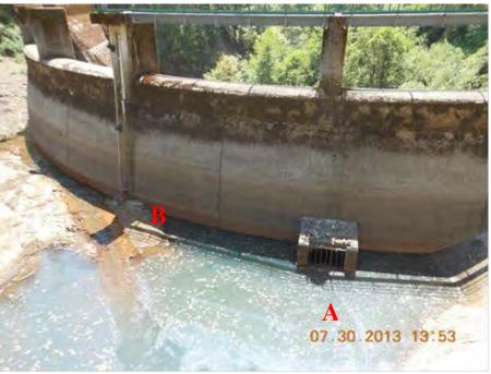
Figure 2.2-14. View to southwest at upstream face of Log Cabin Diversion Dam. The intake for the fish release valve is marked by an "A;" the location of the intake valve stem for the low level valve is marked with a "B."
