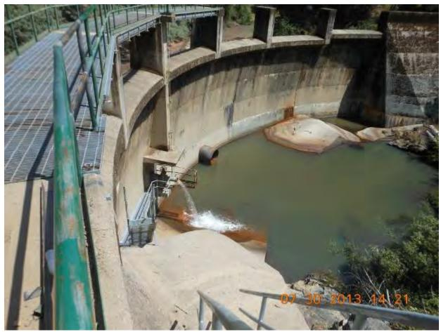
Figure 2.1-1. View to the east of the downstream face of Log Cabin Diversion Dam. The majority of discharge shown in the photograph is through the fish release valve. The low level outlet valve is to the right of the fish release valve.
