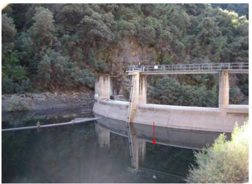
Figure 2.2-17. View looking south at upstream face of Our House Diversion Dam. The inlets for the low level valve and the fish release valve are located below the operator, as indicated by the arrow.
