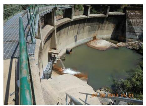
Figure 2.2-13. View to the east at downstream face of Log Cabin Diversion Dam. The majority of discharge shown in the photograph is through the fish release valve. The low level outlet valve is shown to the right of the fish release valve.
