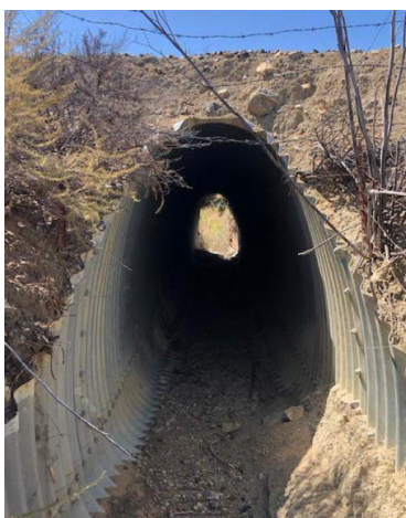
Figure 5: Culvert undercrossing
