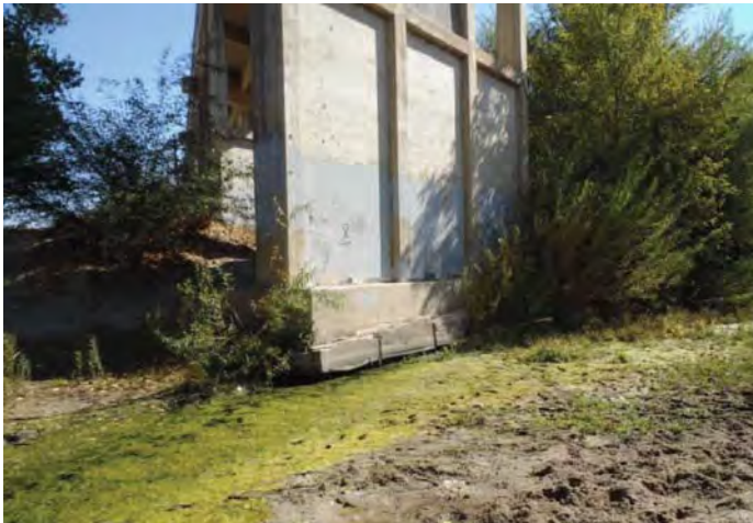
Exposed and Undermined Footing Cap at Bent 19.
