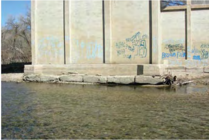
Exposed and Undermined Footing at Pier 18 (Span 17 Side).
