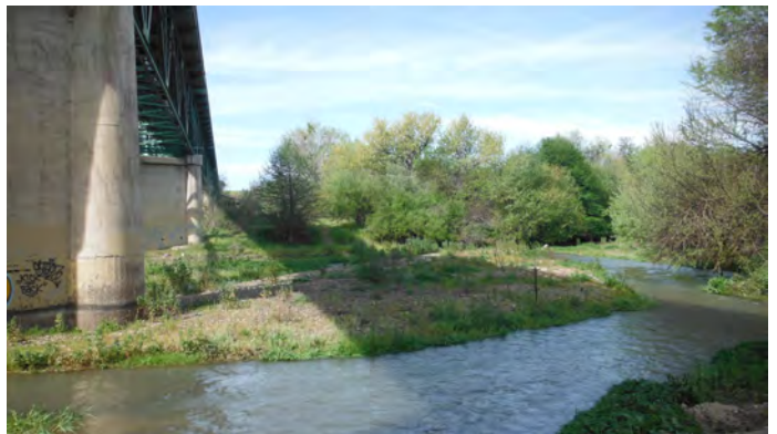
Exposed and Undermined Footing at Pier 17.
