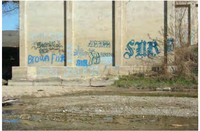
Exposed and Undermined Footing at Pier 19 (Span 18 Side).
