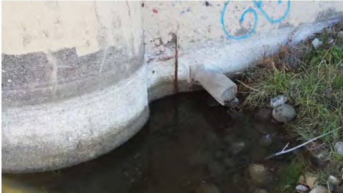
Exposed and Undermined Footing at Pier 16.
