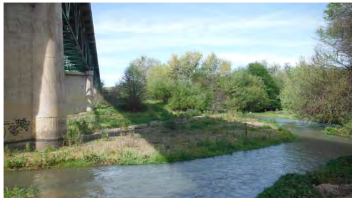
Exposed and Undermined Footing at Pier 17.
