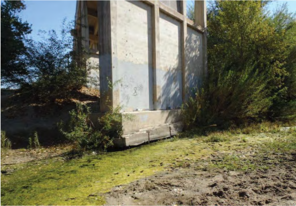
Photo 3. Exposed and Undermined Pile Cap Footing at Bent 19 (Span 18 Side) (10/16/2013)
