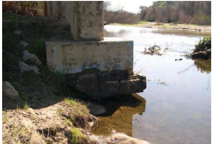
Exposed and Undermined Footing Cap at Pier 19.
