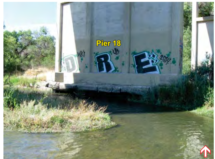
Photo 12. The Salinas River and scour damage at Pier 18, facing north. Photo taken on May 28, 2015.
