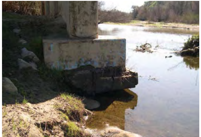
Exposed and Undermined Footing Cap at Pier 19.
