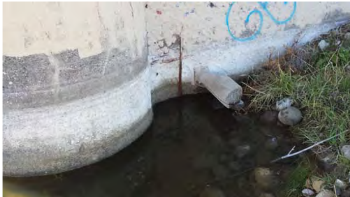
Exposed and Undermined Footing at Pier 16.
