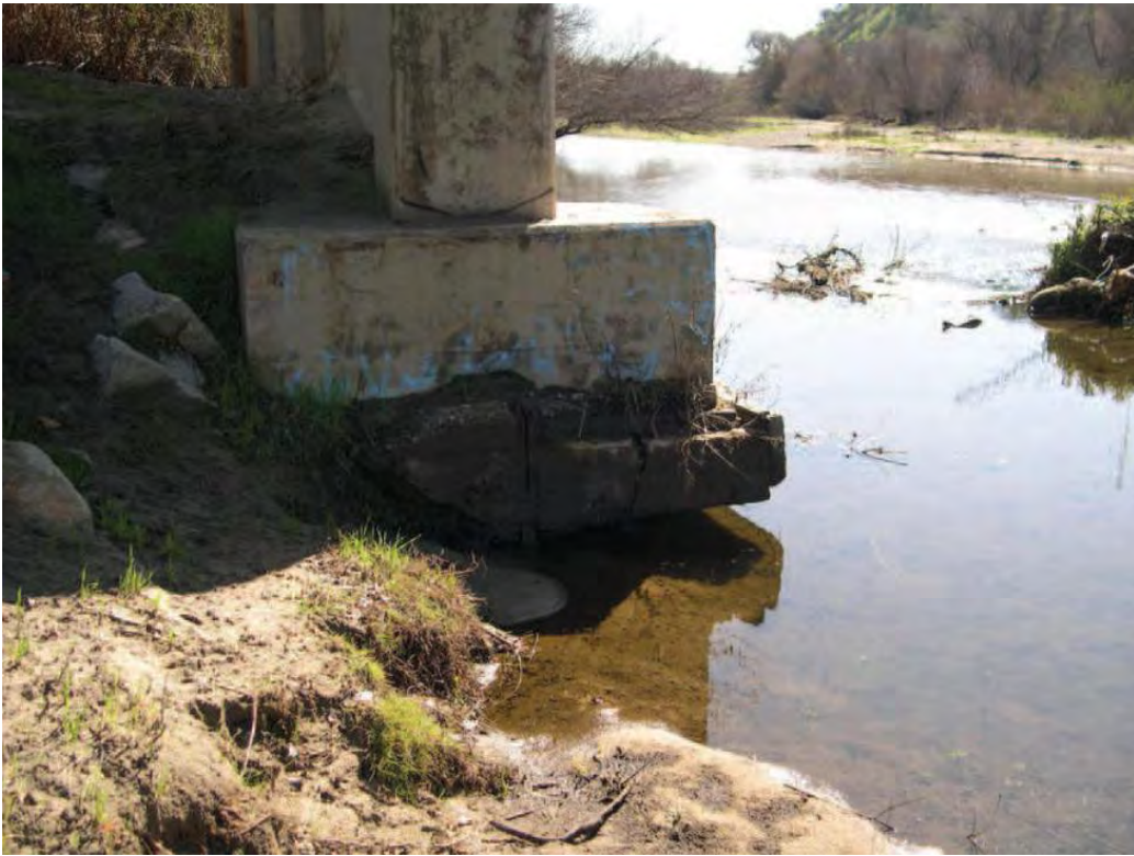
Photo 4. Exposed and Undermined Pile Cap Footing at Pier 19 (02/18/2009)
