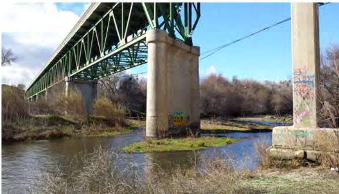
Exposed and Undermined Footing at Pier 17.
