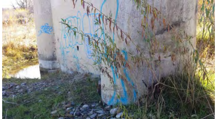
Exposed and Undermined Footing at Pier 16.
