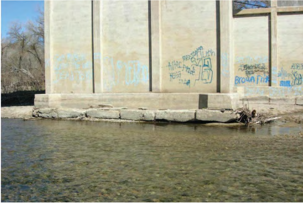
Photo 1. Exposed and Undermined Footing at Pier 18 (Span 17 Side) (02/14/2007)
