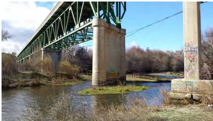
Exposed and Undermined Footing at Pier 17.
