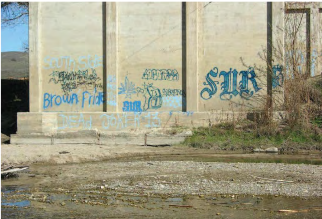
Photo 2. Exposed and Undermined Footing at Pier 19 (Span 18 Side) (02/14/2007)
