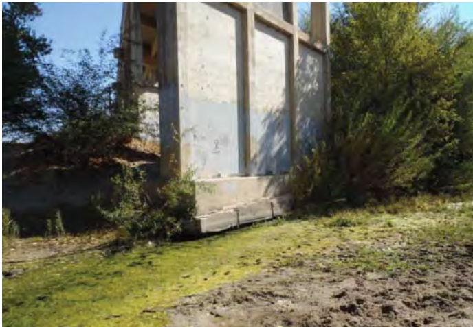
Exposed and Undermined Footing Cap at Bent 19.
