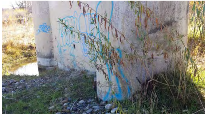
Exposed and Undermined Footing at Pier 16.
