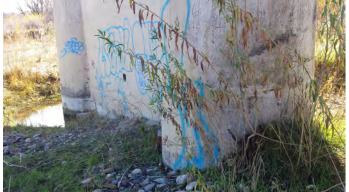
Formation of Scour Hole at Pier 16.
