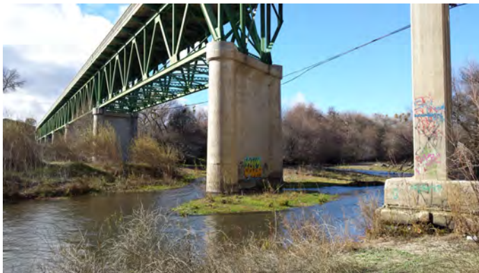
Exposed and Undermined Footing at Pier 17.
