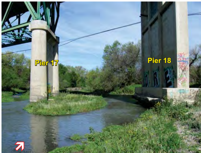
Photo 13. The Salinas River and scour damage at Piers 17 and 18, facing northwest. Photo taken on March 24, 2015.
