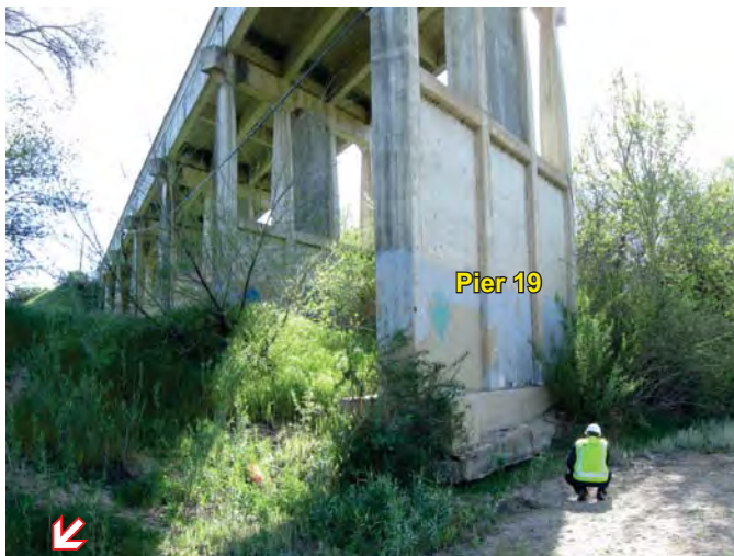
Photo 11. Scour damage at Pier 19, facing southeast. Photo taken on March 24, 2015.
