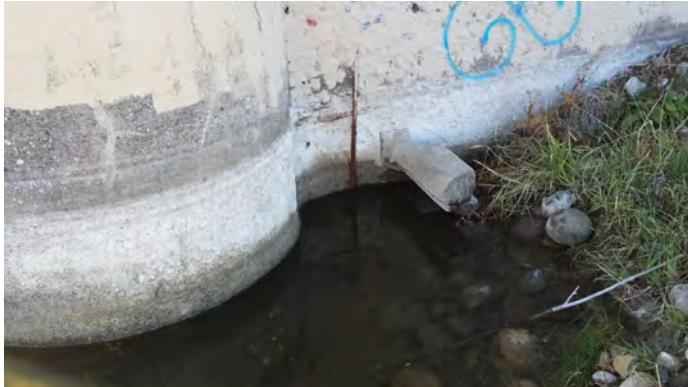
Exposed and Undermined Footing at Pier 16.
