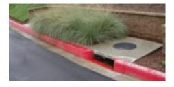
working to break down and remove non-point source pollutants. The flow rate is controlled in the MWS Linear, giving the plants more contact time so that pollutants are more successfully decomposed, volatilized, and incorporated into the biomass of the MWS Linear's micro/macro flora and fauna.
