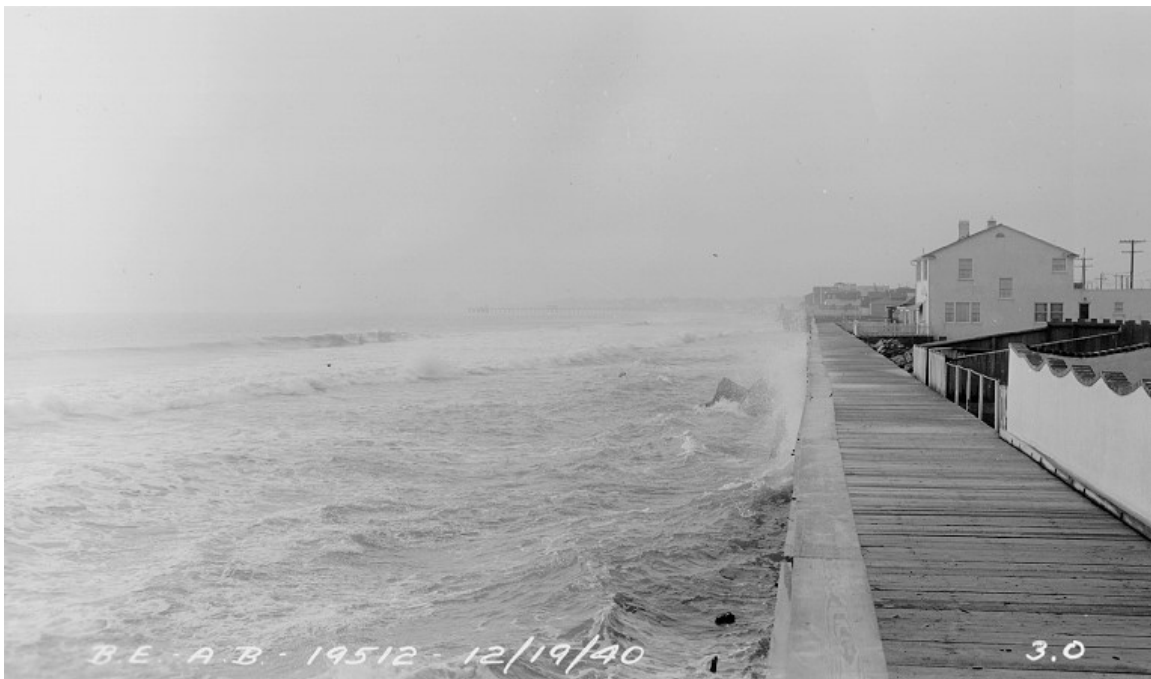
Figure 7-57: Waves impacting the bare timber bulkhead along Peninsula Beach in 1940 without the protection of the Long Beach Breakwater
