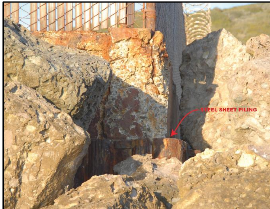
Figure 1-4. Steel Sheet Piling Foundation at Concrete Vault
