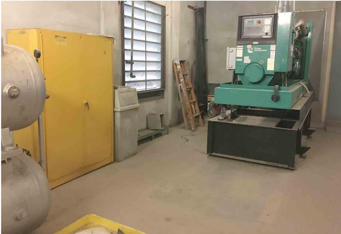
Photo No. 7 Diesel backup generator on the 17th floor
