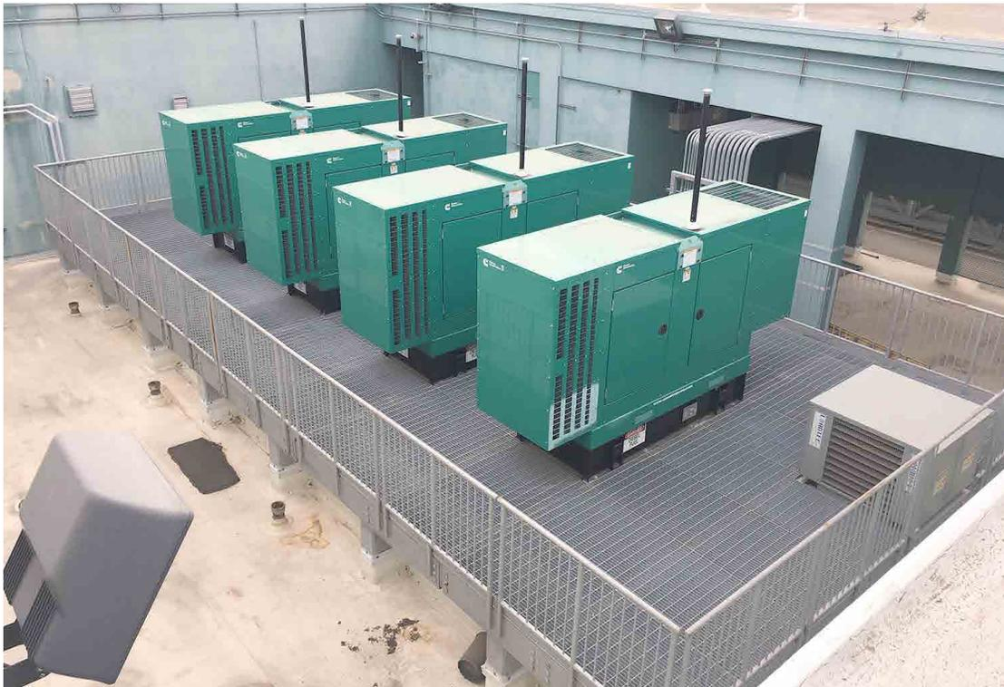
Photo No. 6 Diesel backup generators on the 17th floor
