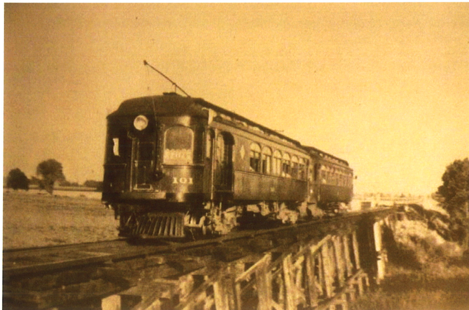
Photograph 4: Sacramento Northern at Marty, 1940. Note that every tenth tie is 10 ft long to carry the third rail. (Photo taken from Swett et al.: 1981:77)
