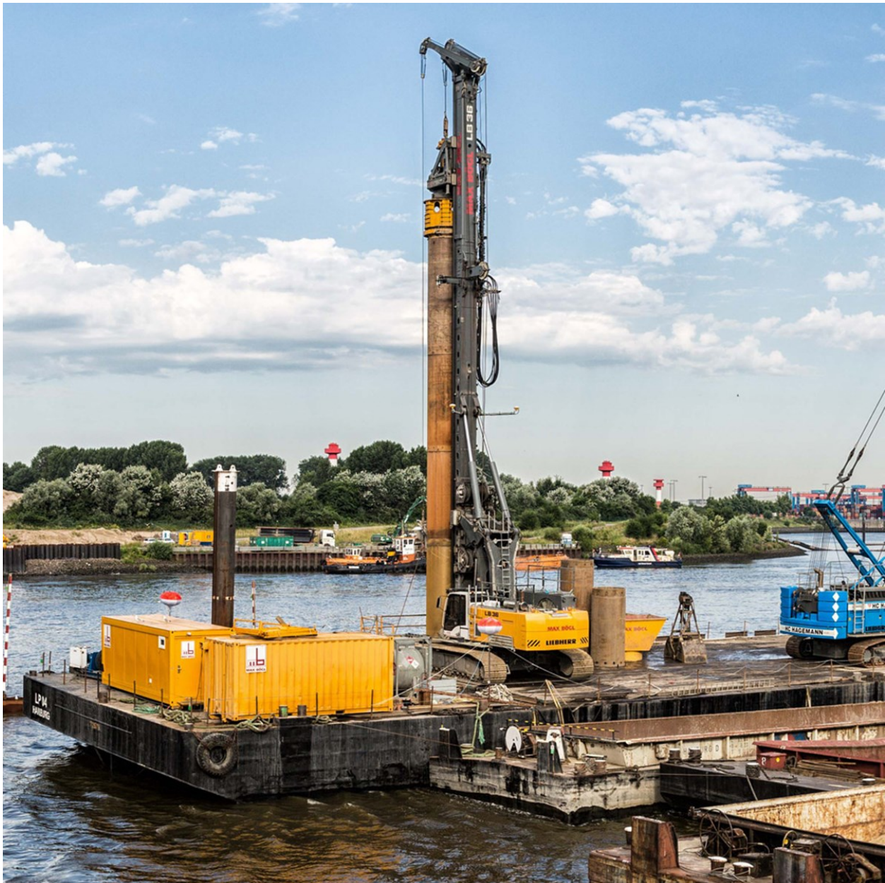
Figure 11. Barge-mounted Rotary Drill Rig
