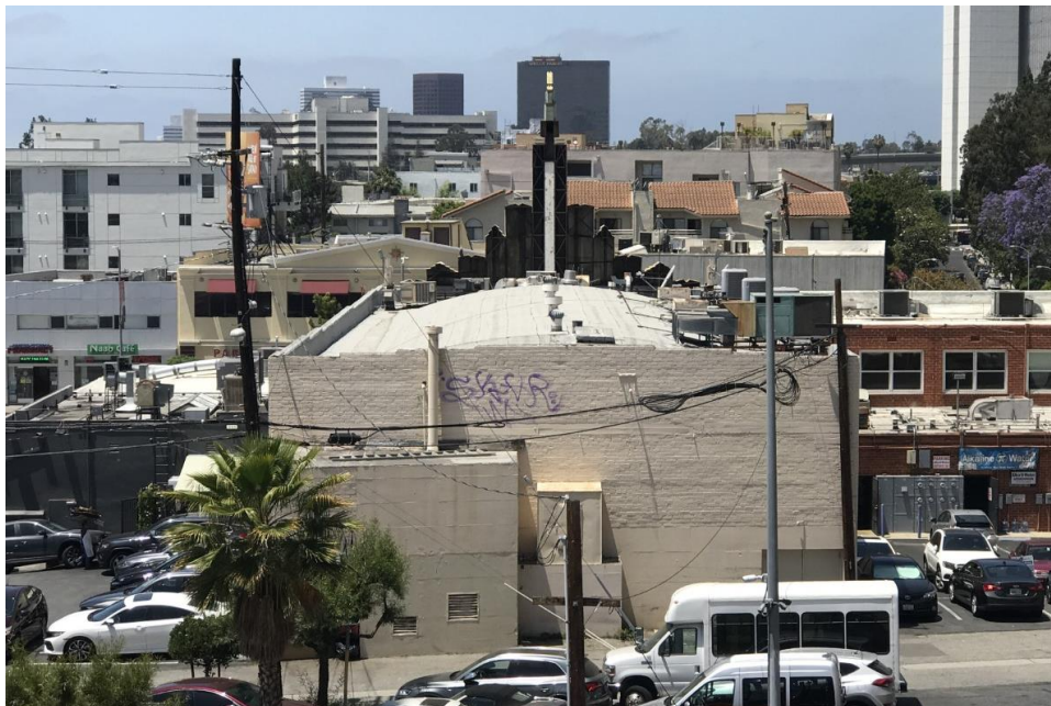
Figure 9: Rear (east) façade, with the bowed truss roof visible as well as the exposed framing of the front (west) upper façade, looking west.
