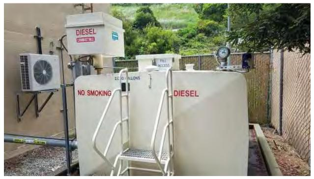
Photograph 8: Generator storage tank on the (adjacent) Comcast property
