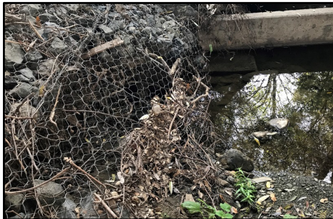
Photo 5: Alpine Road UC (L/R) Bridges; View south east of the gabion mattress (left side) and a weir (upper right side)
