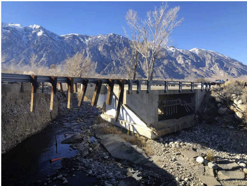
View of existing failed bridge over Pine Creek and abutment to be removed.
