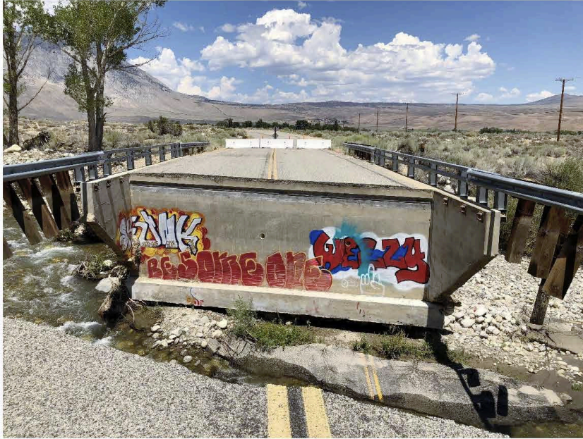
View of existing failed bridge over Pine Creek. A portion of the existing bridge abutment is located within the OHWM of Pine Creek.
