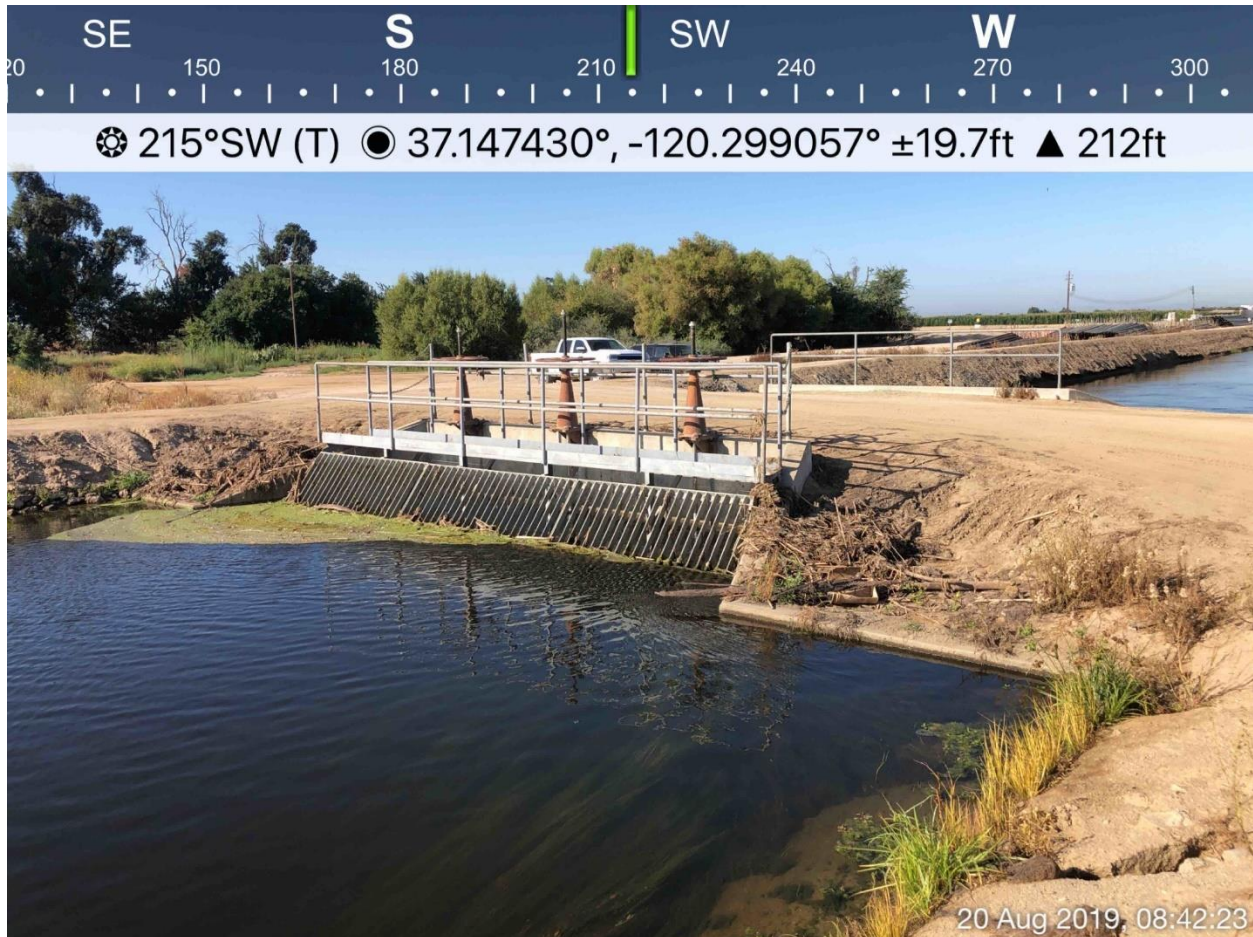
Photograph 18: LaBranza Main Canal “drop.” This is the location where water from Chowchilla River flows into LaBranza Main Canal. Pondweed and algae are visible along the control gates in this photograph.
