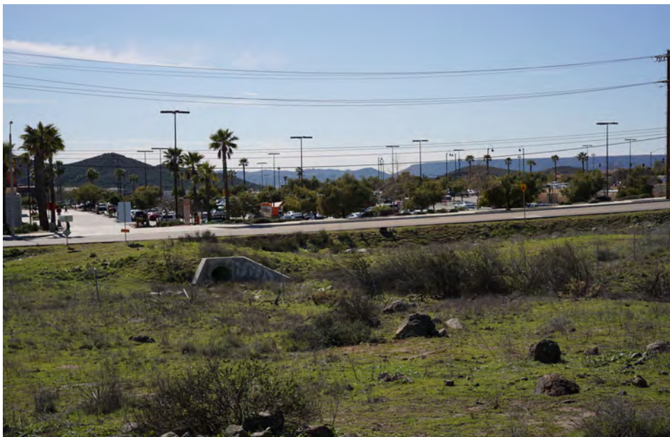
48-inch culvert at the southern portion of the project site where both drainages exit the project area.
