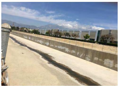
Photo 7. Upstream view of Ordinary High Water Mark data point 1 (OHWM 1) taken within the concrete-lined Cucamonga Creek located just east of the project boundary and survey area. Tenfoot wide low-flow channel estimated by presence of flowing water and staining. 76-foot wide active floodplain estimated based on the flat channel bottom and 5- and 10-year flow events that occur within the full extent of the channel.
