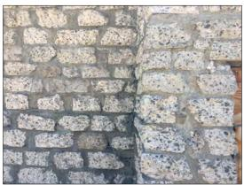
Fig 1 (left): Subject property, west elevation (center) and south façade (right), view northeast (McGee, 2019); Fig 2 (right): Subject property, west elevation, detail of concrete rubble exterior wall material, view west (McGee, 2019)
