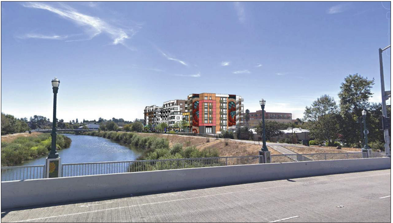
Looking Southwest From Soquel Avenue Bridge
