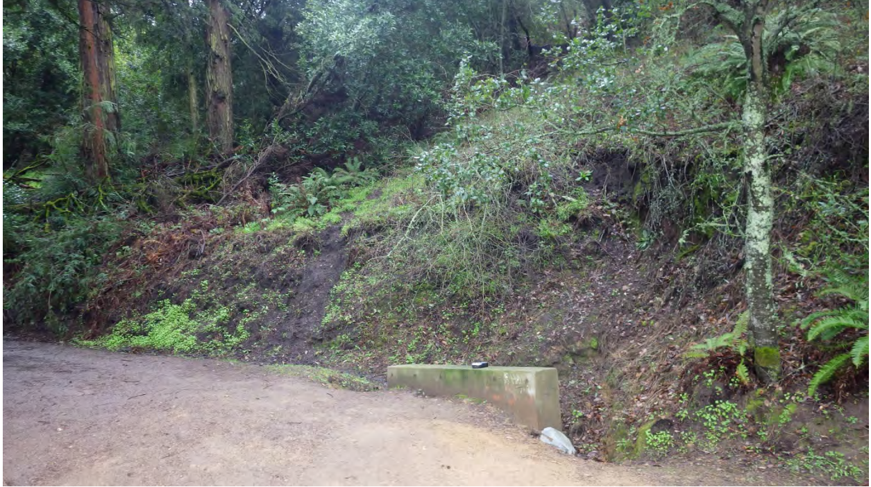
Photo 1. Drainage moves into culvert and beneath road.
