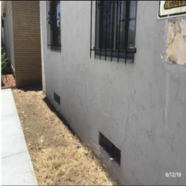
View of Stucco over Stud Walls
