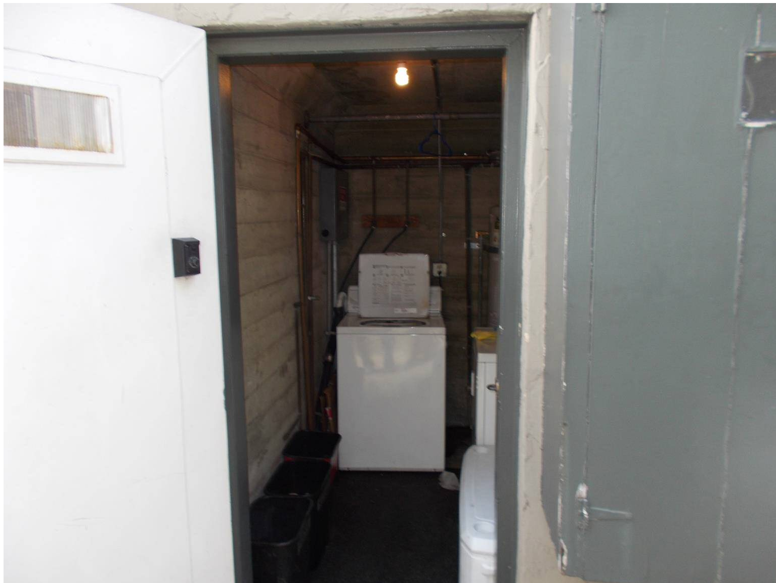
DSCN3694 Washer is used for oily rags from the trucks and uniforms. Washer also leaks water on floor.
