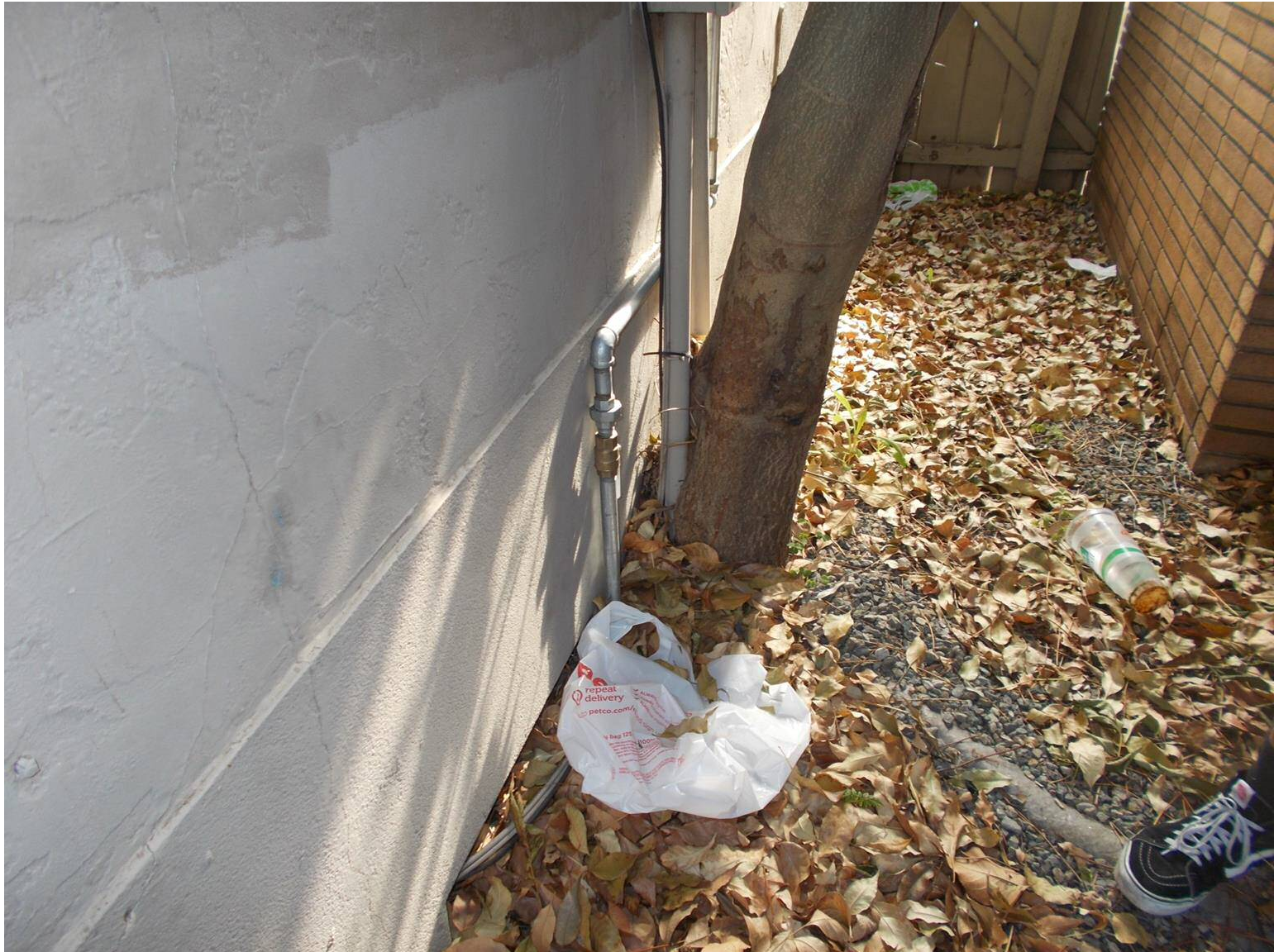
DSCN3700 Tree growing out of the building and around piping.
