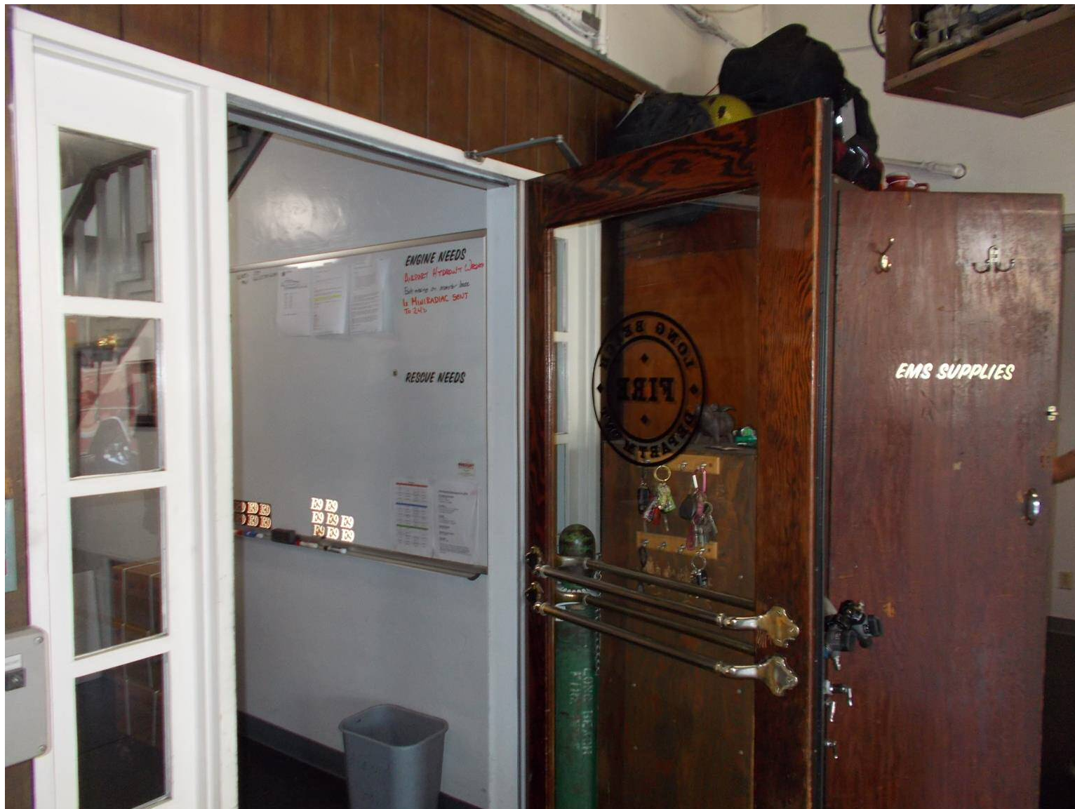
DSCN3687 It is questionable whether this is a proper door between the garage and the living spaces of the station.
