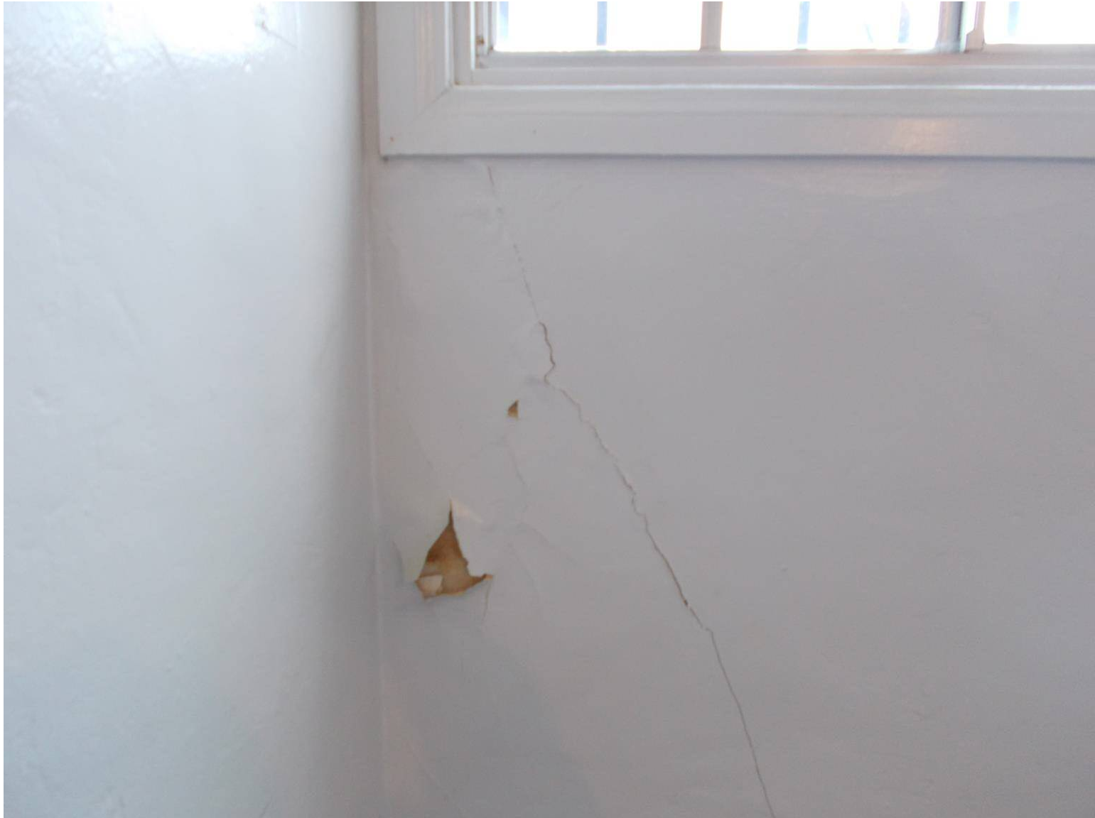
DSCN3651 Delaminated paint and cracks in stairs.
