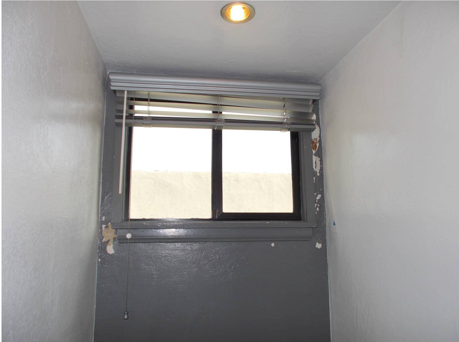
DSCN3659 Areas around 2 nd Floor Bedroom #3 window paint is delaminating and cracks observed. Area is falling apart.
