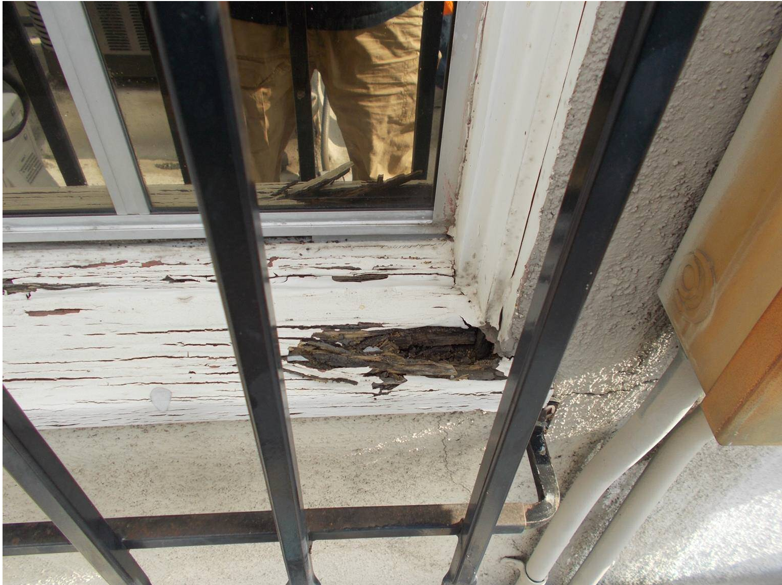
DSCN3653 Window frames are dry rotted and falling apart. Possible reason for blistering paint and cracks in stairs
