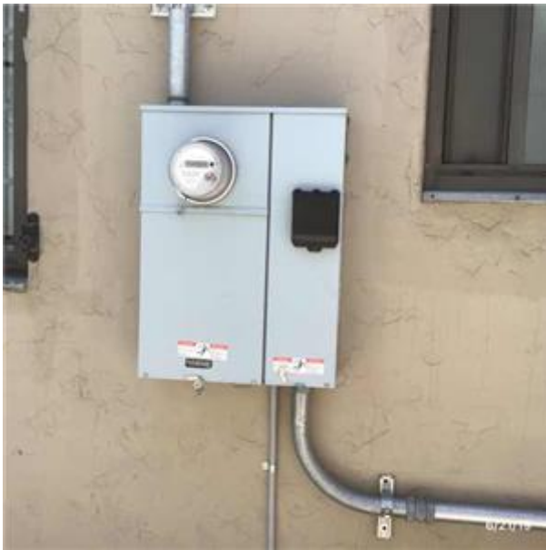
View of Panelboard - 120/240volts, 60 to 2000amp
