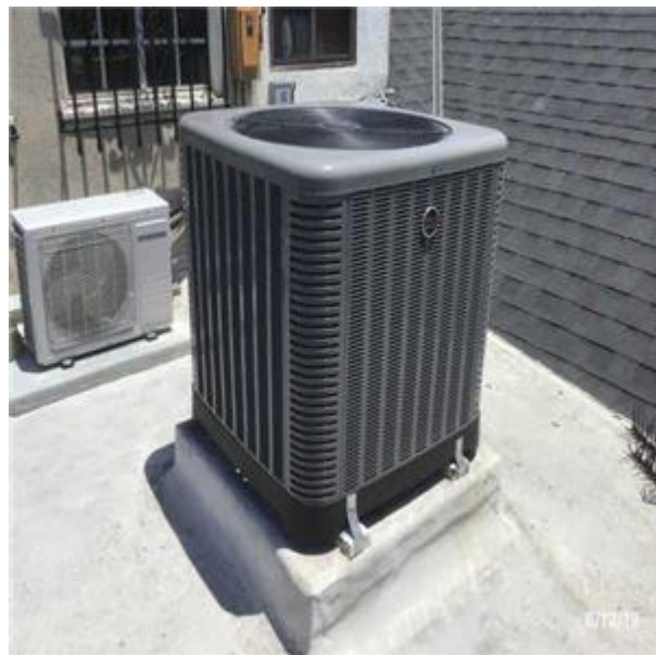
D3032 Direct Expansion Systems :- View of Split-System (Full System)
