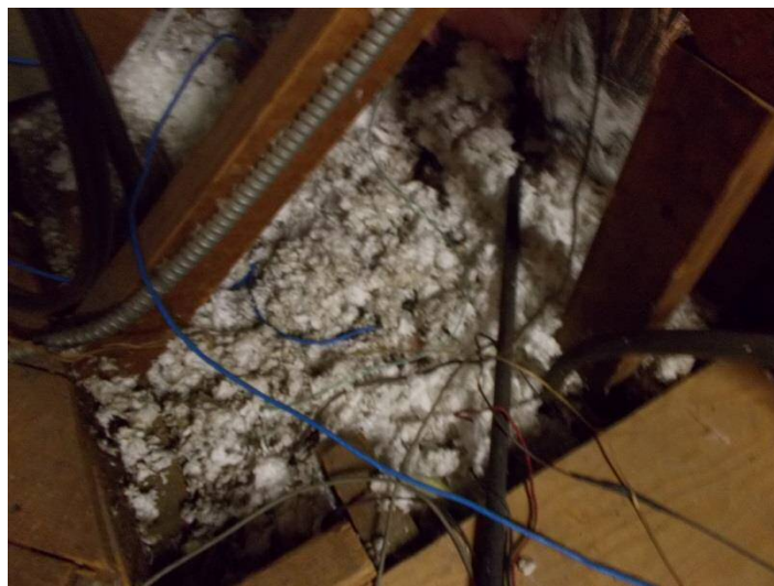
DSCN2654 Attic Insulation (Concern whether or not it contained Asbestos), Records Research to be Conducted
