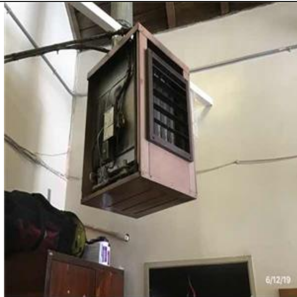
D3051 Terminal Self-Contained Units :- View of Unit Heater - Gas Fired Suspended - 20 MBH
