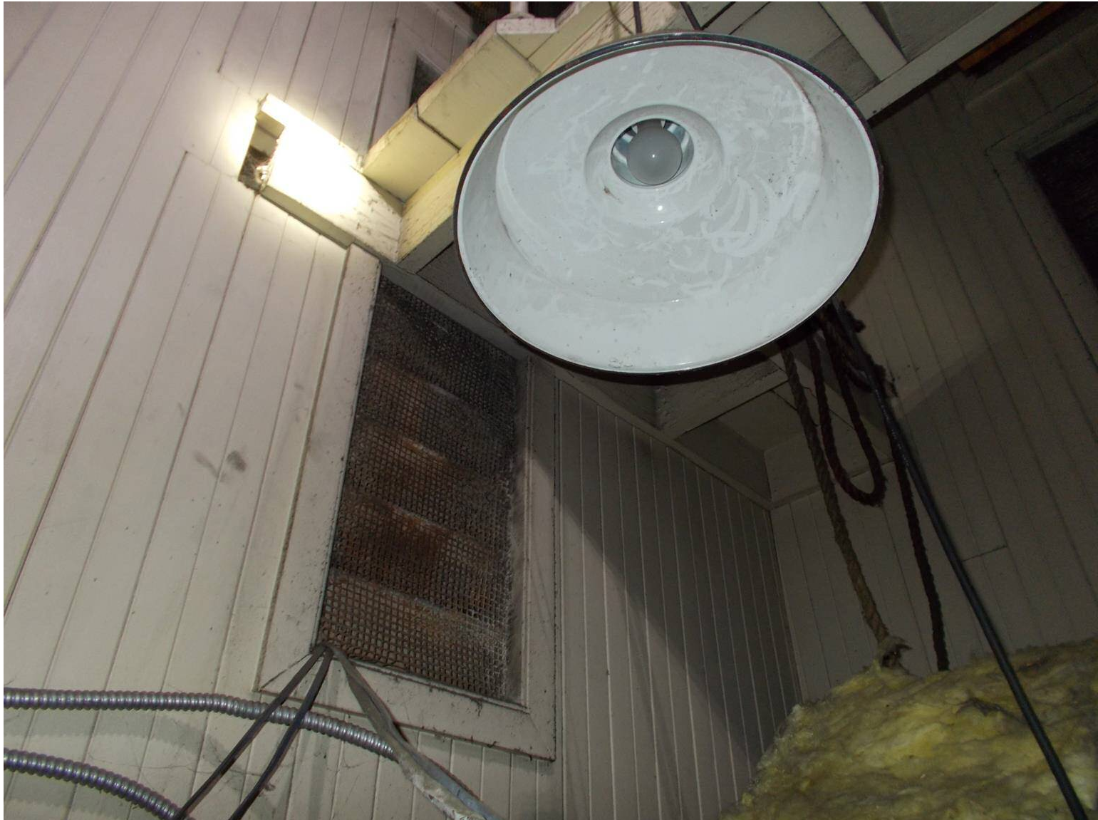
DSCN3665 Bedroom is not sealed from outside. Vents are open.
