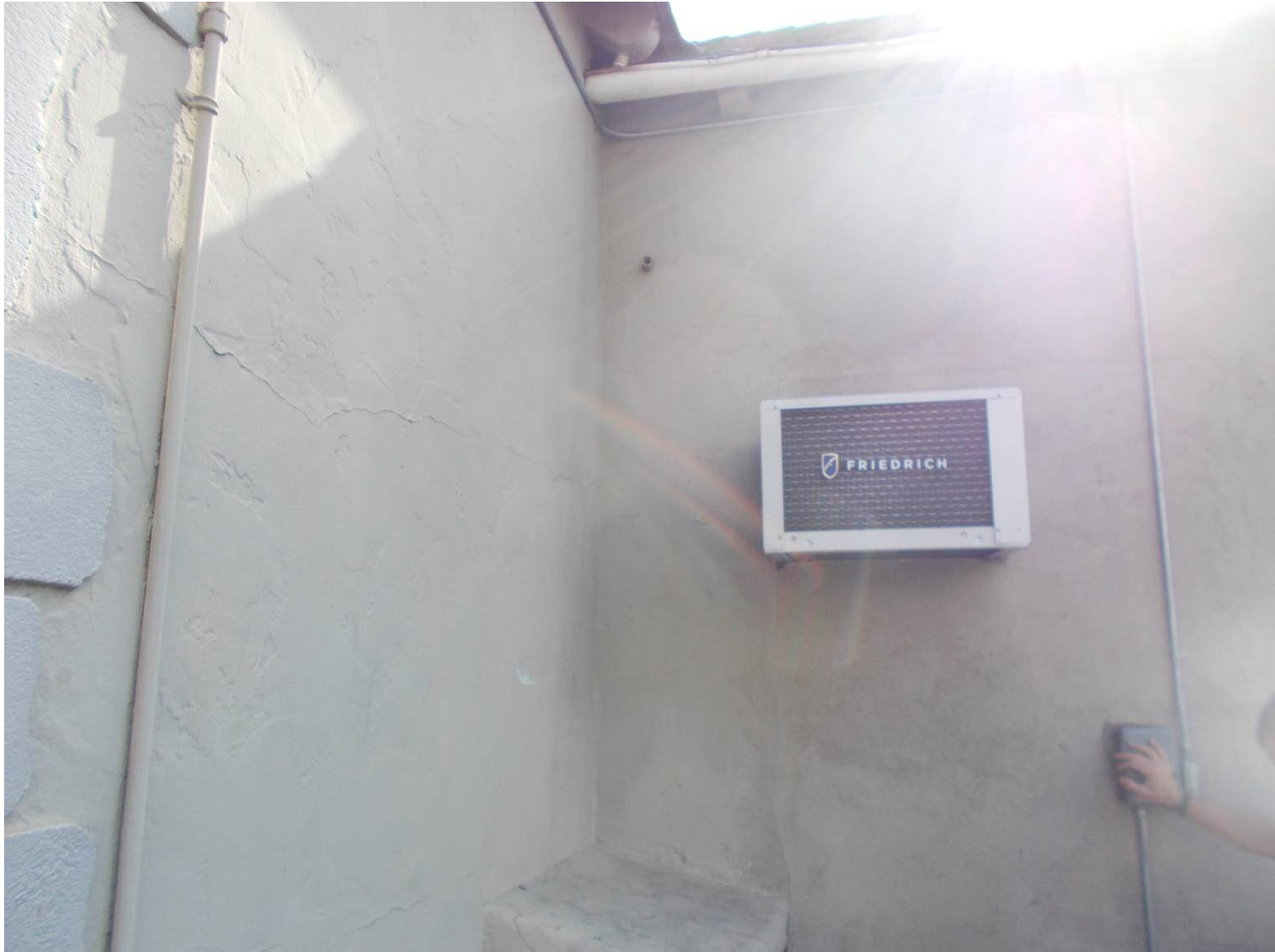
DSCN3697 Wall mounted HVAC unit 1 st floor has gaps.
