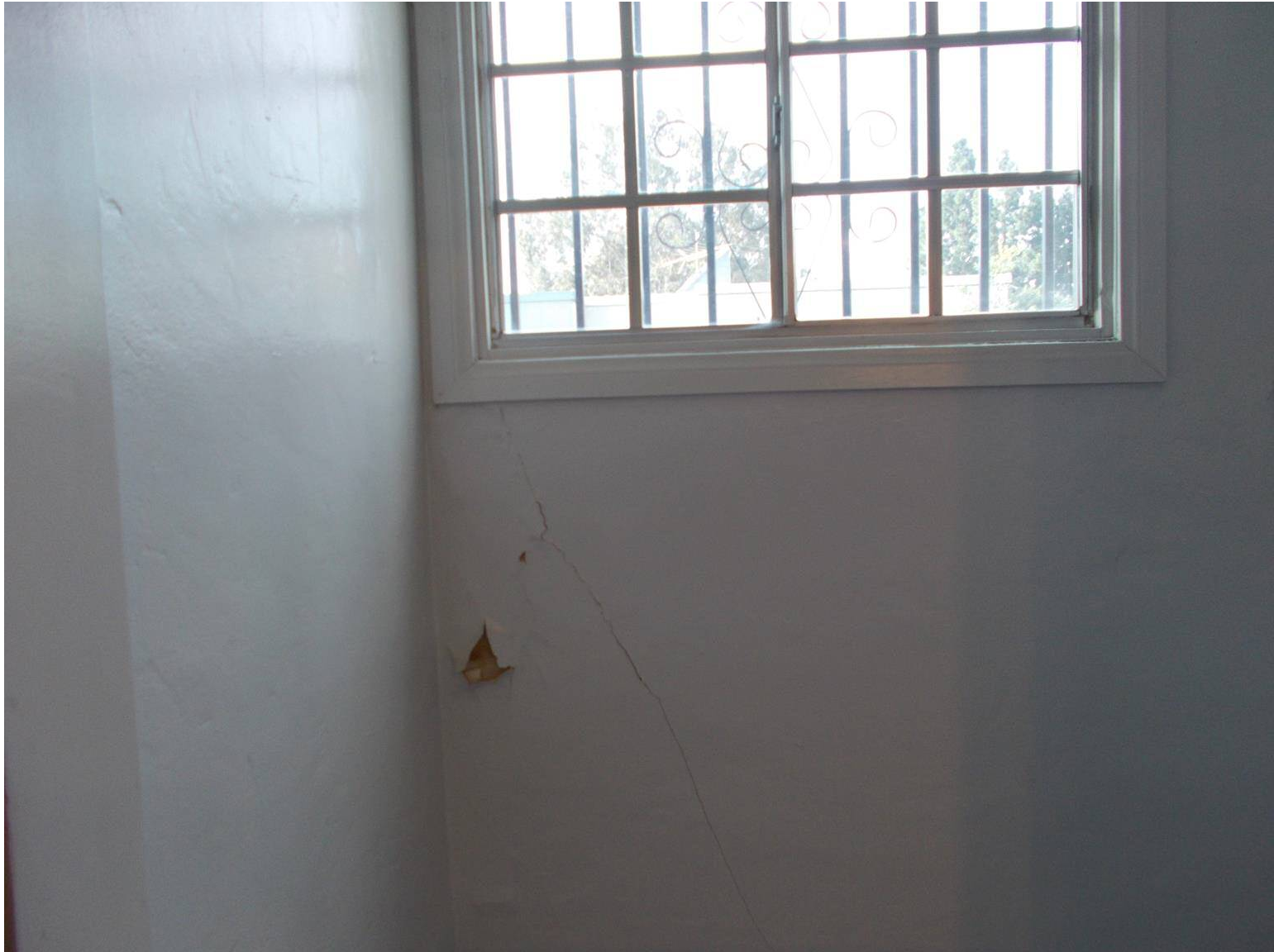
DSCN3650 Delaminated paint and cracks in stairs.
