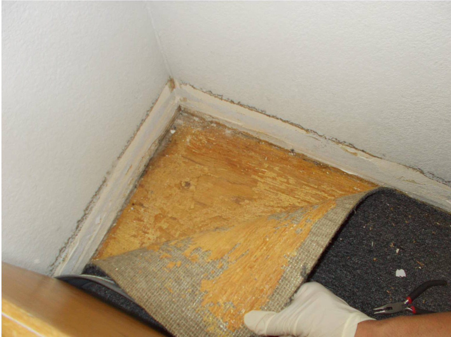
DSCN3810 2 nd Floor, Bedroom #1 Inspection around "Leaking Windows."
