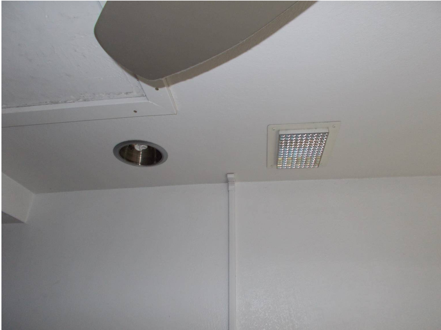
DSCN3674 Dust and gases migrate from light canister, access hatch, and vent(s) in bedroom at the ceiling.
