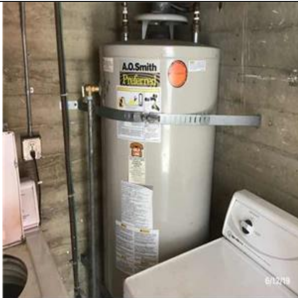
View of Domestic Hot Water Heater - Gas
