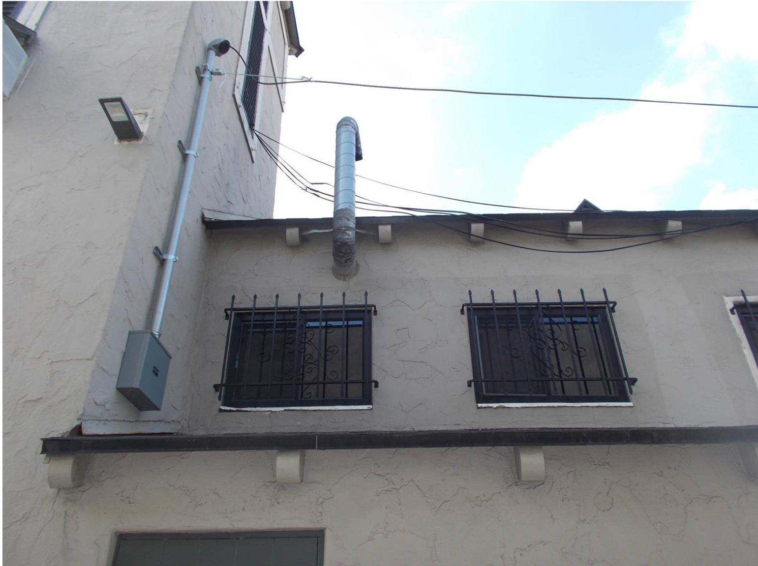
DSCN3691 The distance between the exhaust (truck exhaust system) and the open louvers in the hose tower is close.
