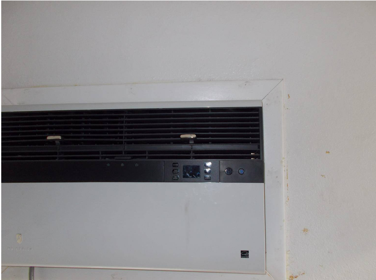
DSCN3675 Wall HVAC unit gaps where you can see the outside.
