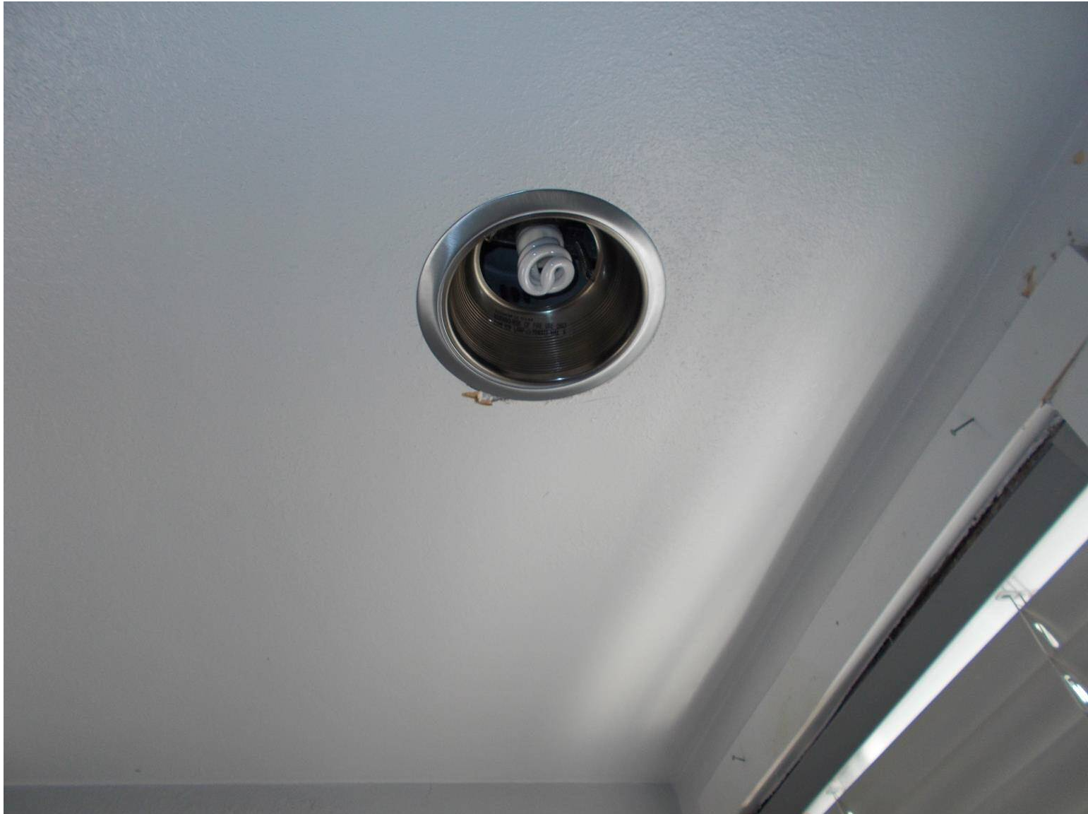
DSCN3676 Can light where dust and gases can migrate into the bedroom from the hose tower.
