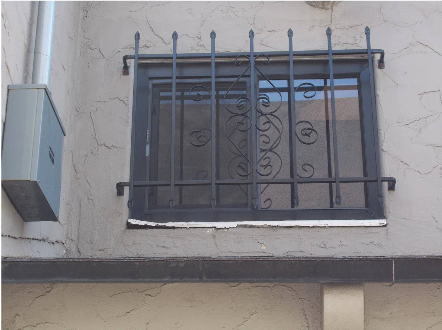
DSCN3693 Framing around window is deteriorated.
