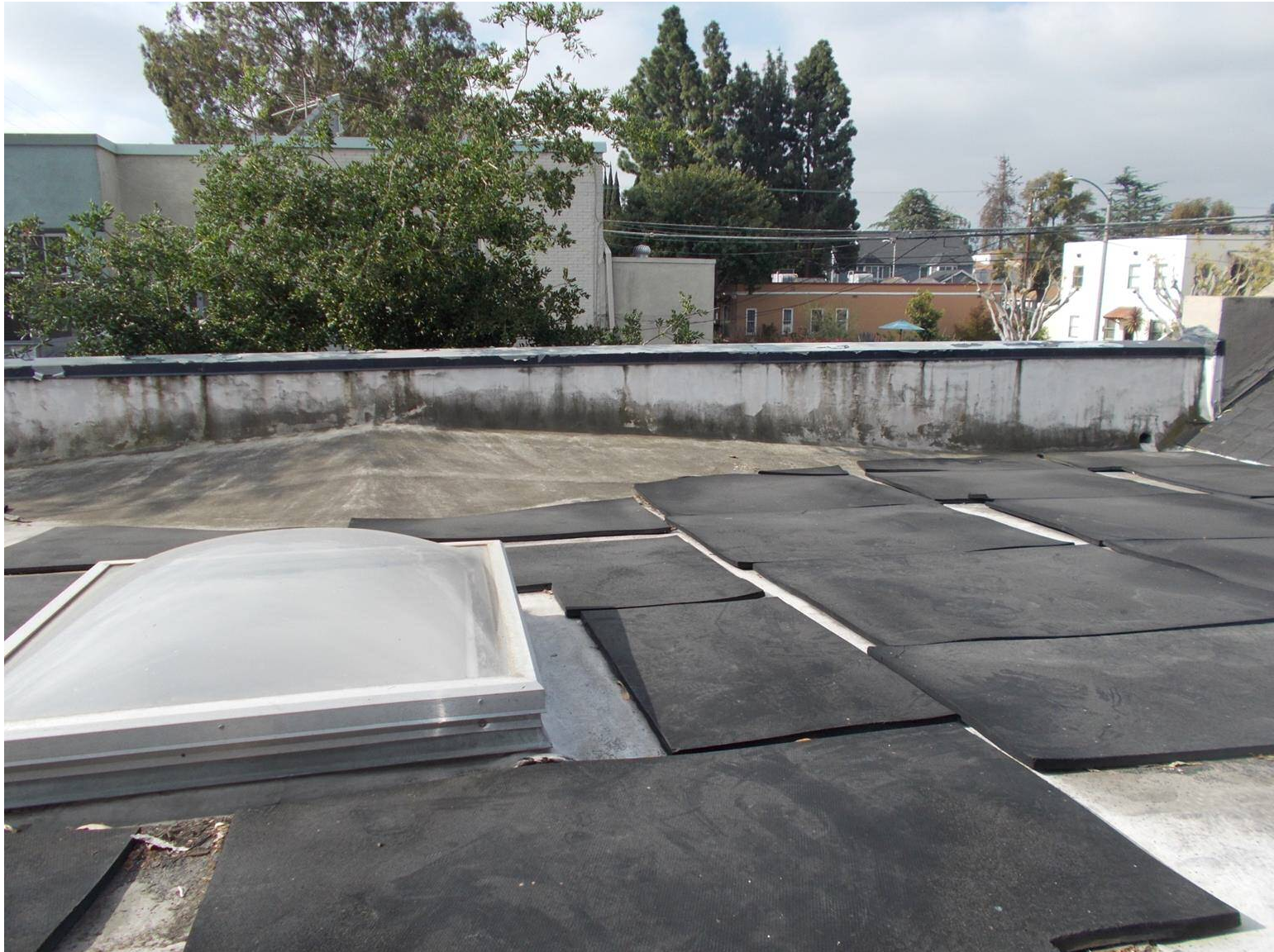
DSCN3662 Dark stains are observed around parapet and is believed to be mold.
