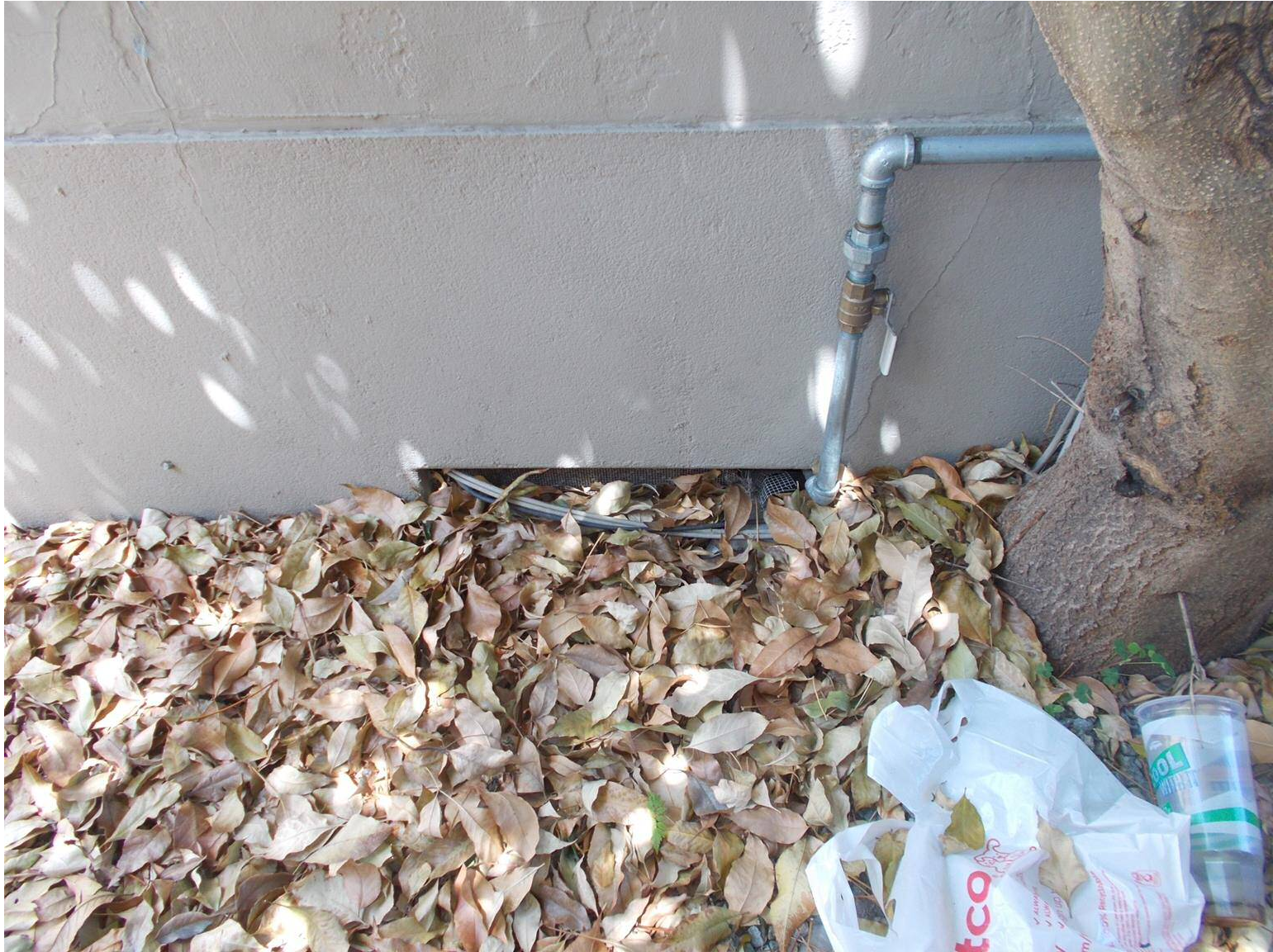
DSCN3869 Inspection of building perimeter. Crawlspace vent clogged with leaves.
