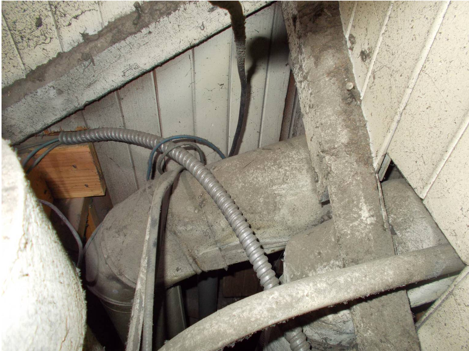
DSCN3669 There are gaps which lead into the garage where gases can migrate in and eventually settle in the bedroom.
