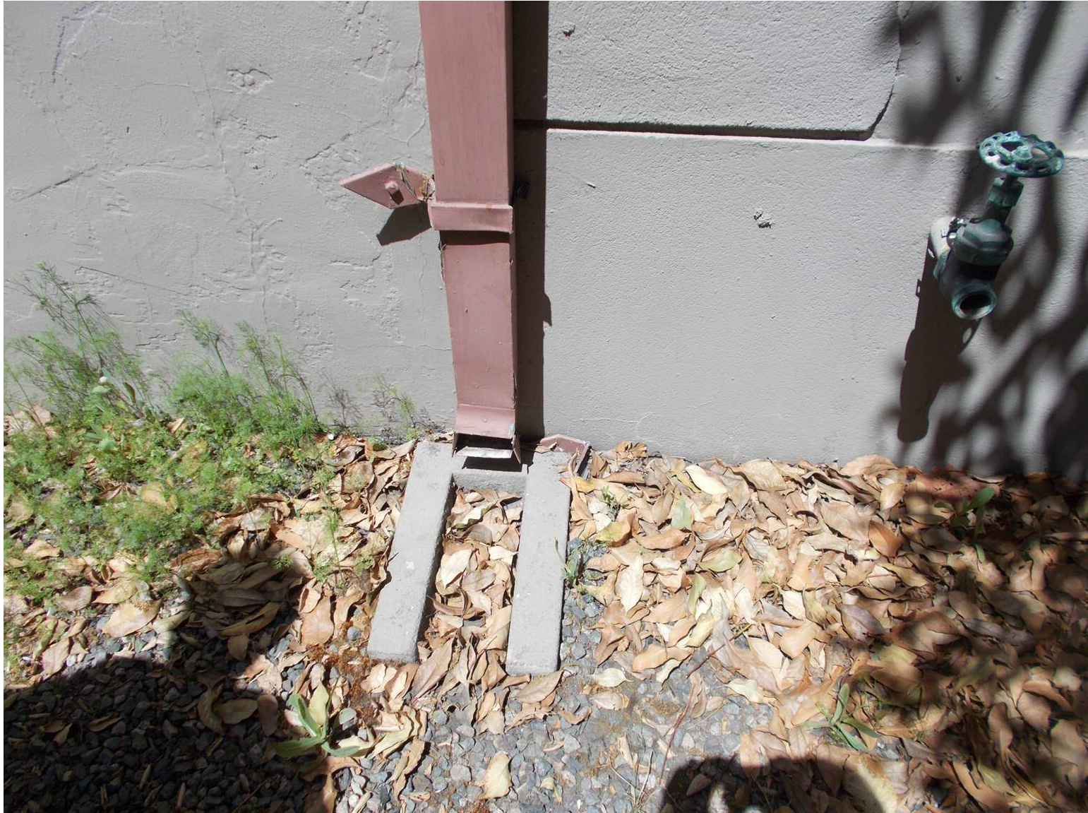
DSCN3873 Holes in building not sealed. Drainage not correct.
