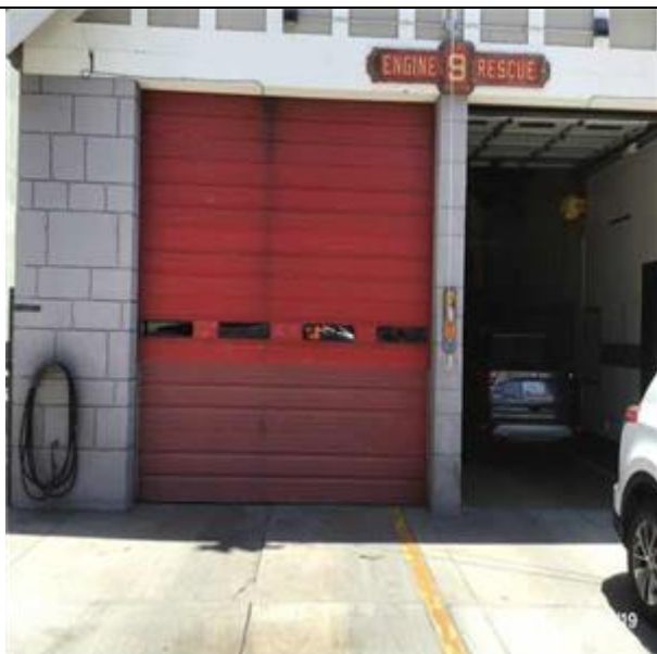
View of Rolling Overhead Doors, Electric
