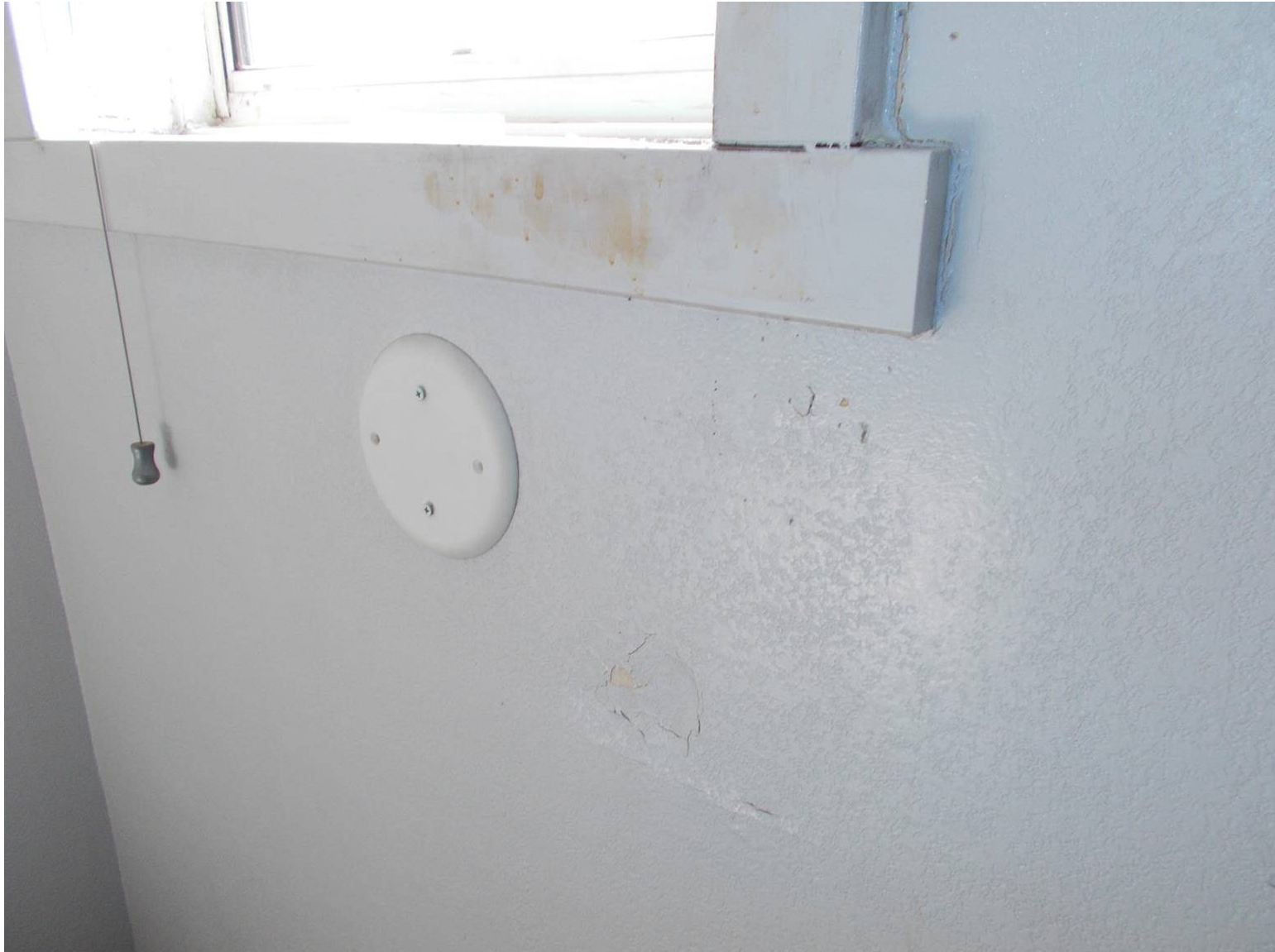
DSCN3679 Paint is blistered and cracks are observed. Water stains on sill are observed.
