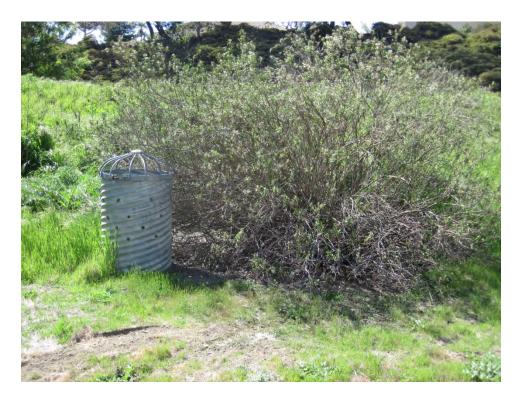
Photo 10. View of the standpipe at the west end of the swale which appears to transmit storm water to storm drain system.
