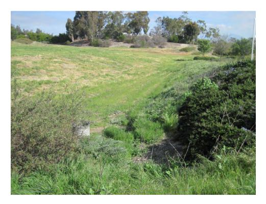
Photo 8. View of the swale which appears to collect storm water sheet flowing over study area to prevent it from running into parking lots and buildings (standpipe in foreground).
