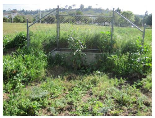
Photo 4. View of concrete inlet which appears to collect runoff from adjacent manufactured/landscaped slopes between the study area and residential development.
