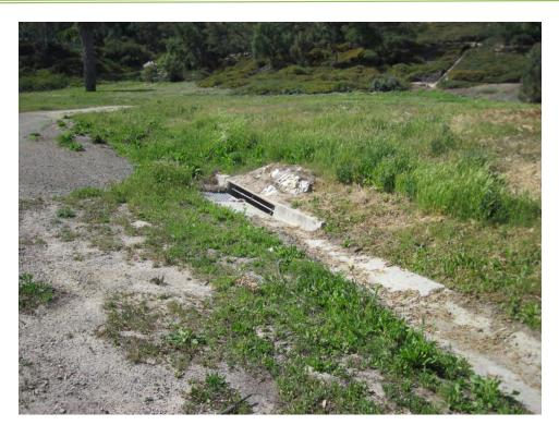
Photo 7. Typical storm drain and concrete feature adjacent to on-native grassland.
