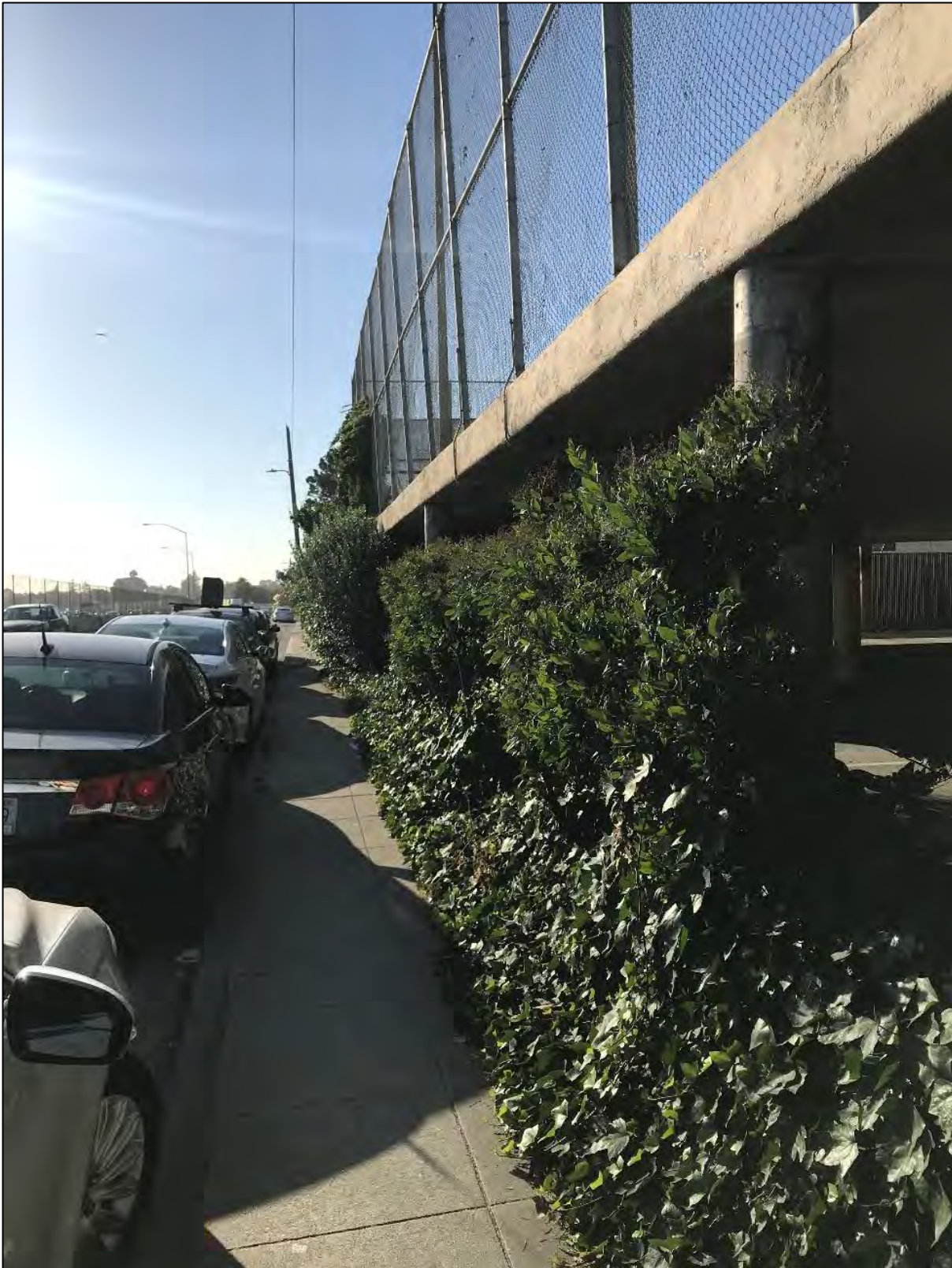
Photograph 1. Shrubs to the north of the tennis court, facing east.
