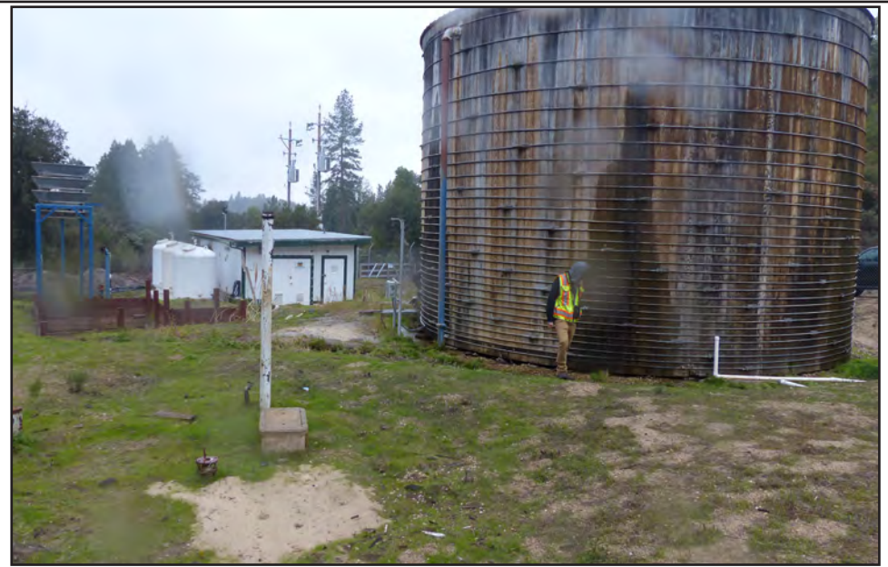
Photo 2. View of Lewis tank site looking south, showing the existing leaky redwood tank and abandoned water treatment infrastructure.
