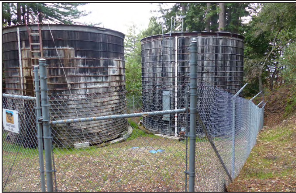
Photo 1. View of Kaski tank site looking southwest, showing the existing leaky redwood tanks.
