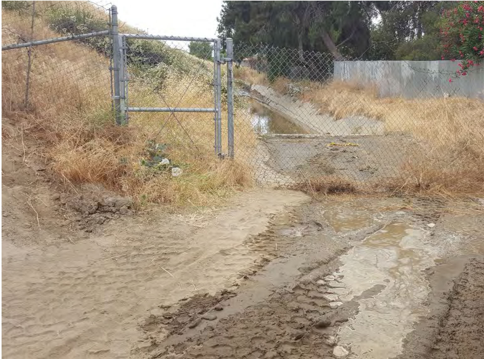
Figure 11: 66" CSP Outlet Basin West of Interstate-15
