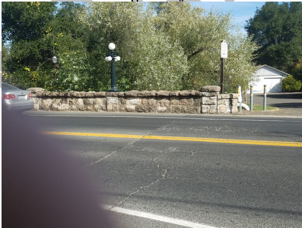
Northbound side bridge rail. 8" PG&E gas line (White) behind bridge rail.
