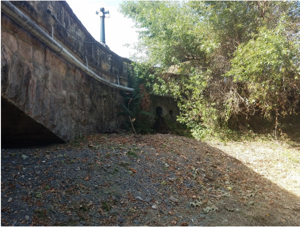
Northbound side of Sulphur Creek. Right wall abutment has 2 outfall culvert pipes. PG&E gas line strapped to bridge.
