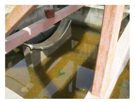
Photo # 14: showing secondary containment of diesel tank containing liquid. As per Gerry Ruiz this is rainwater.
