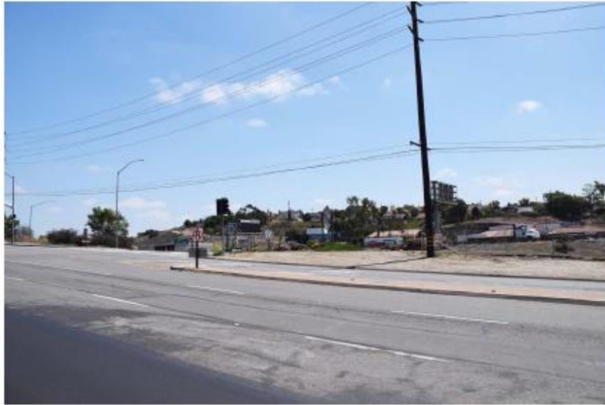
SB SR 55 off-ramp: This view looks towards the Lincoln Ave. SB SR 55 off-ramp at N Tustin St.
