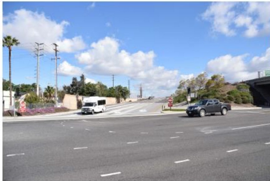
Visual simulation of the proposed roadway widening. In this view, an additional lane is added to the SB SR 55 Katella Ave. off-ramp and the storm drain is relocated to beyond the proposed inside shoulder.
