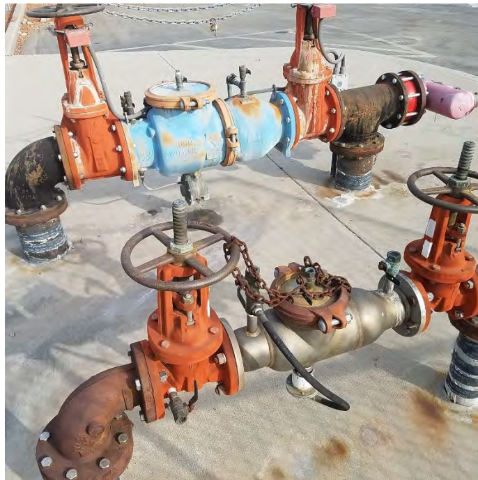
Photograph 6: View of water meter and control system adjoining the south of the site. The water pipeline is six inches in diameter.
