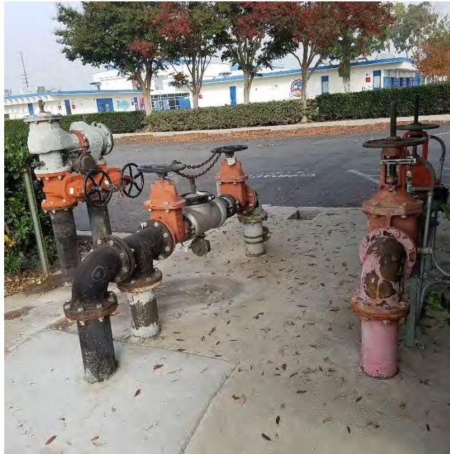
Photograph 5: View of water meter and control system adjoining the south of the site. The water pipeline is six inches in diameter.
