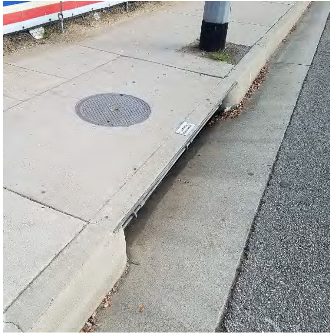
Photograph 3: View of a stormwater catch basin on the sidewalk of Cerritos Avenue to the southwest of the site.
