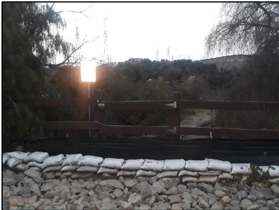
Photograph 4. Detail of erosion barrier
