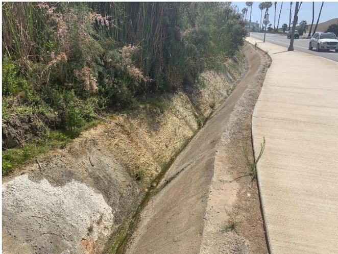
Photo 8: Superior Avenue wetlands. Note excess water draining off slope into the concrete-lined drainage ditch at toe of slope.
