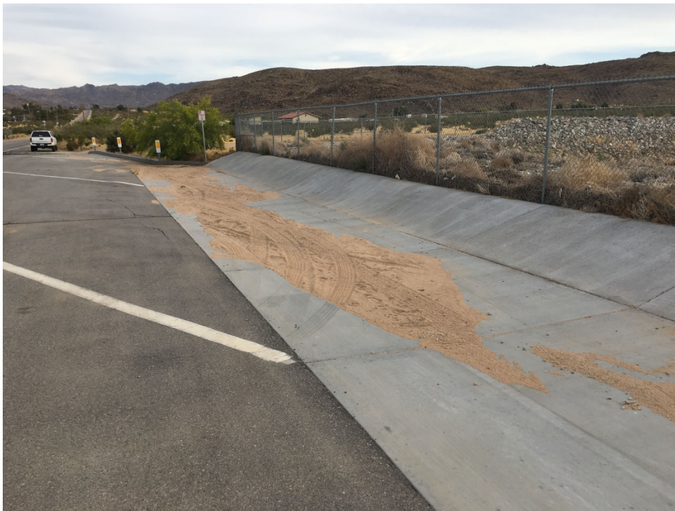
Photo 16: Retention Basin Overflow
