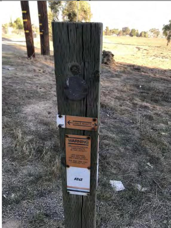
A secondary fiber optics pole nothing the west/east direction of the cable route
