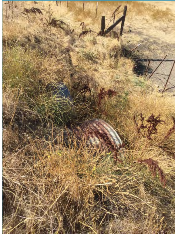
Photograph 7. Feature I, an ephemeral feature conveyed under Avenue 26 via two 24" CMPs, facing northwest.
