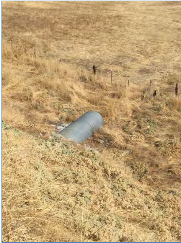
Photo 3: View of typical culvert conveying small amounts of ephemeral flow under Road 29.
