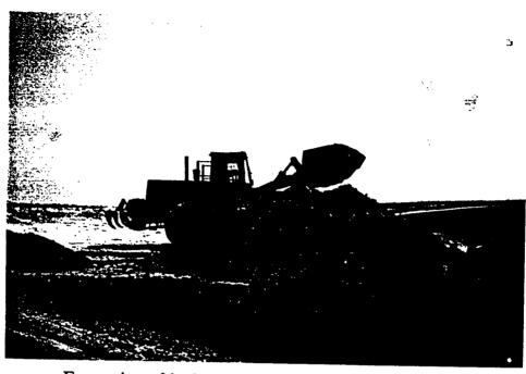
Excavation of hydrocarbon stained soil at Well #2-10.
