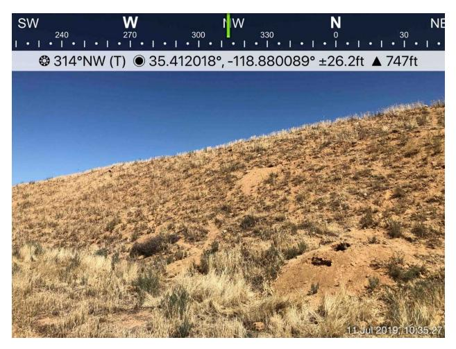
Photograph 12: Overview of one of the large earthen berms onsite. Both berms were riddled with burrows.
