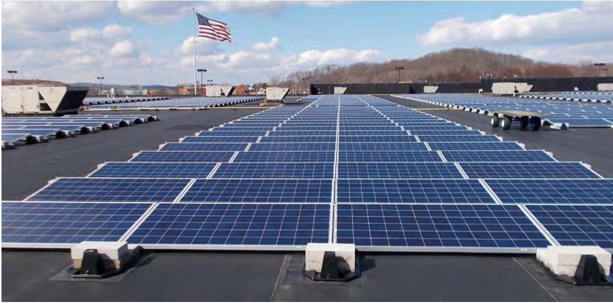
Typical Roof Mounted “Self-Ballasted” Solar System
