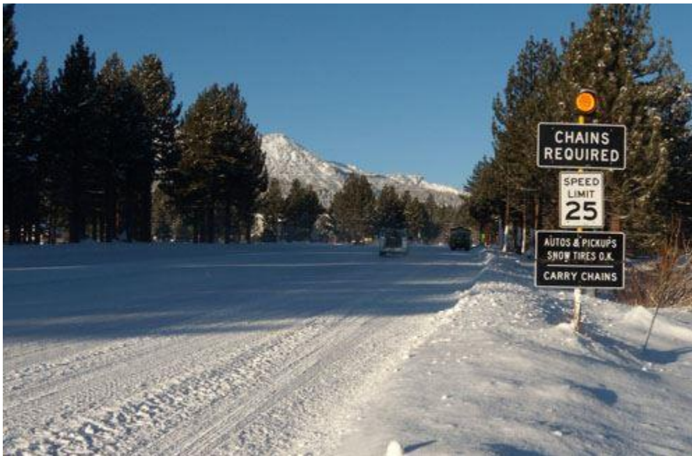
Figure 3 - Example of an existing chain control sign with attached flashing beacon. Due to updating sign standards, new signage proposed in this project will likely be similar but may not exactly match this image.
