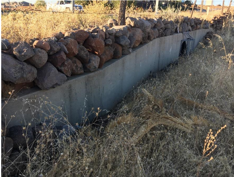
Figure 2D: Headwall and trash guard at outlet for C1B
