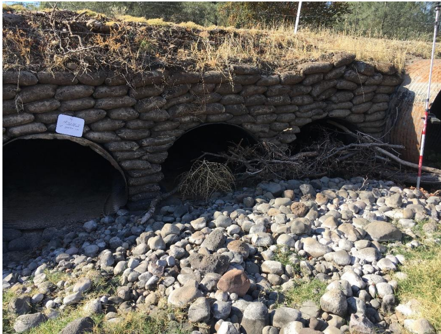
Figure 7A: C6 Culverts inlet with obstructing branches
