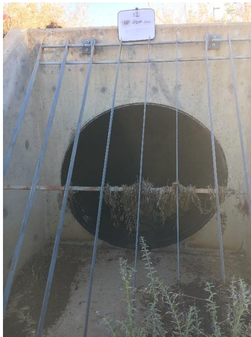
Figure 2A: Headwall and trash guard at inlet for C1A
