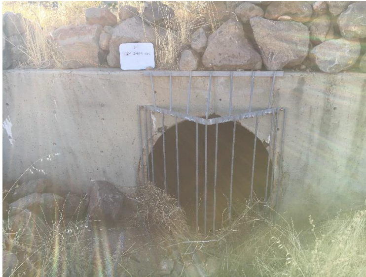
Figure 2B: Headwall and trash guard at outlet for C1A
