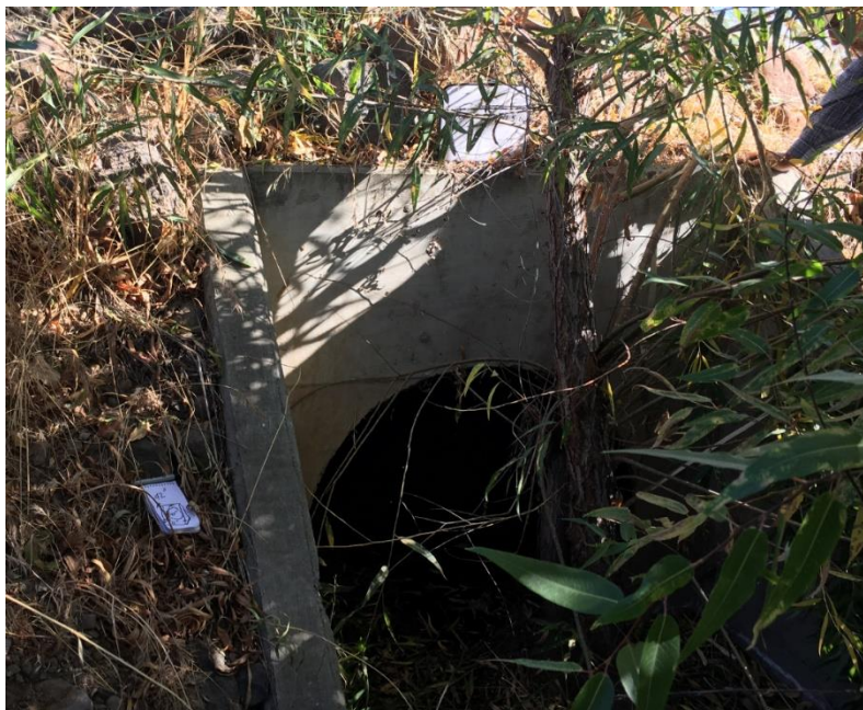
Figure 2C: Headwall and trash guard at inlet for C1B
