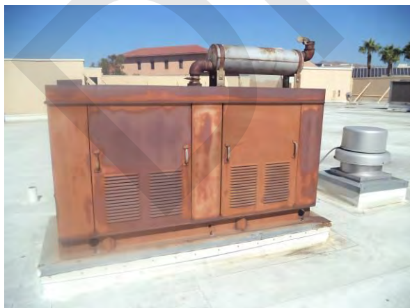
Photo #35 View of natural gas powered emergency generator located on the north side of the roof.
