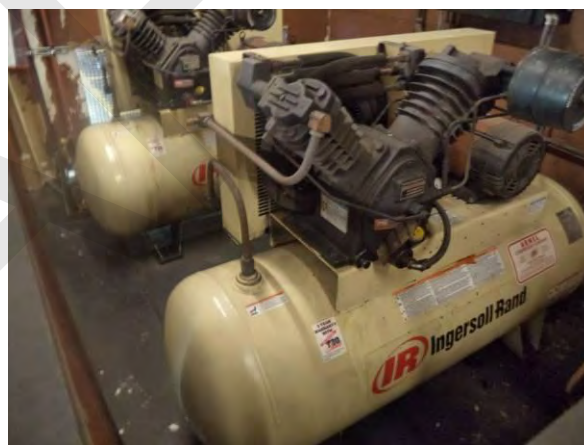
Photo #16 View of two air compressors located in automotive service center on southwest side of site.
