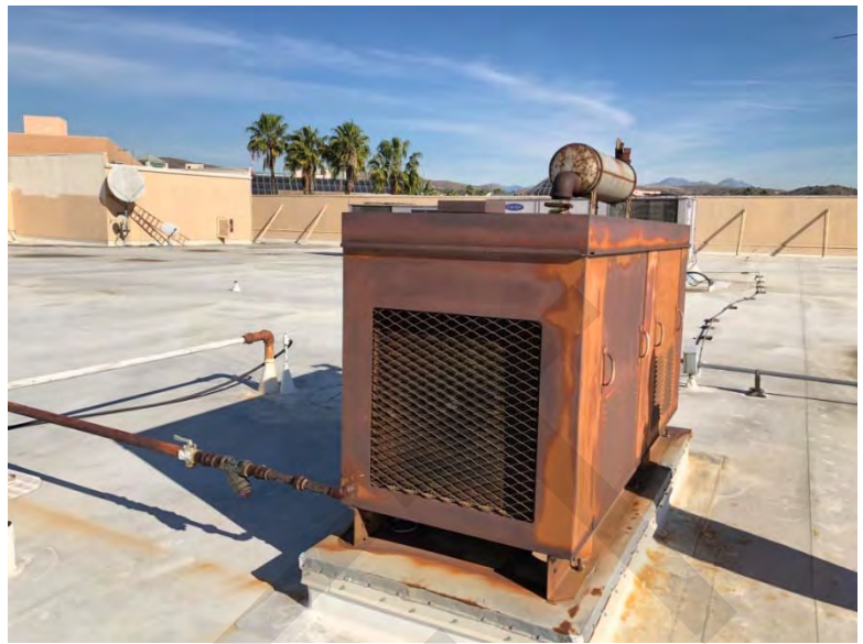
Photograph 16: Gas-fired emergency generator on roof
