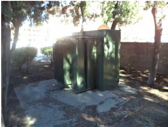
Photo #37 Typical view of pad-mounted transformer located on northwest side of site.
