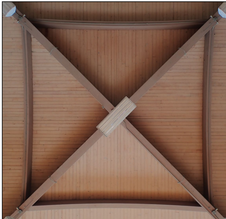
War Memorial Community Center. Barrel groin vault roof. View south. 3/19/19.
