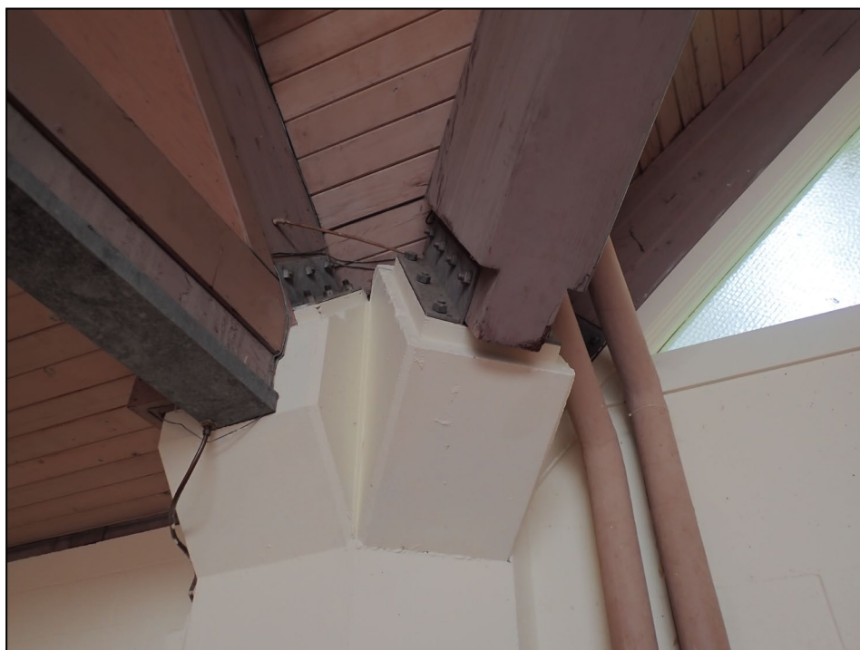
War Memorial Community Center. Second floor basketball court. Groin vault roof beam support detail. View west. 3/19/19.
